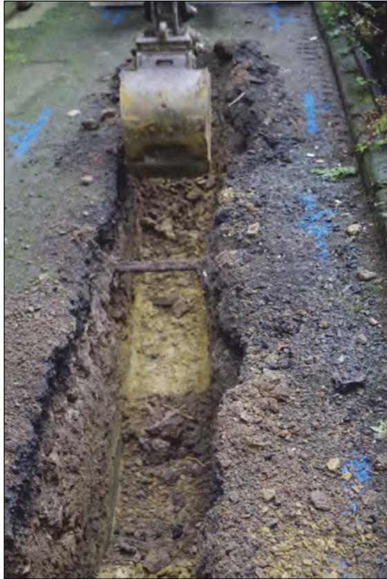
Plate 1: Excavation of Trench 1
