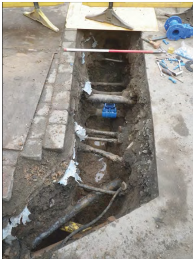
Plate 4: Overview of Trench 2
