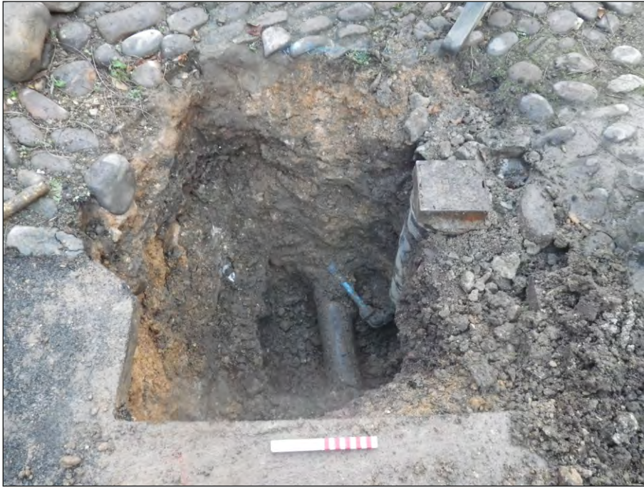
Plate 1: Trench 7 in Heritage Zone 1, camera facing east
