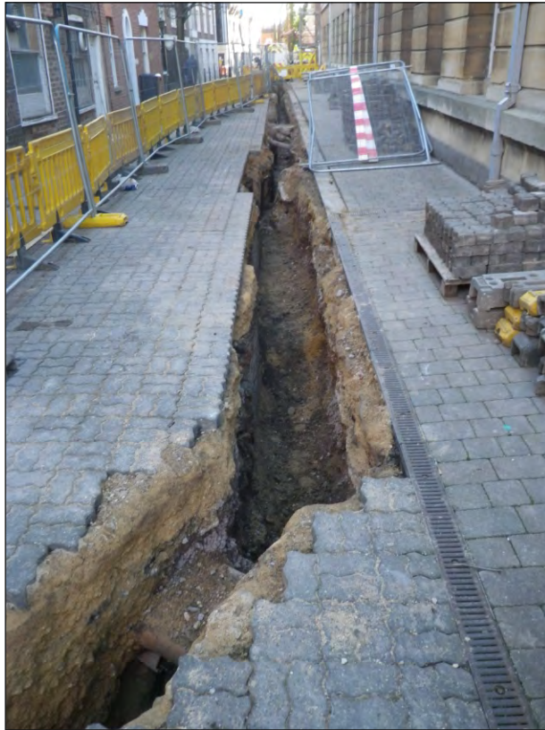
Plate 27: General view of trench 80 in Heritage Zone 9, camera facing south-west
