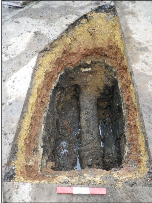
Plate 31: Trench 178 in Heritage Zone 10, camera facing south-west
