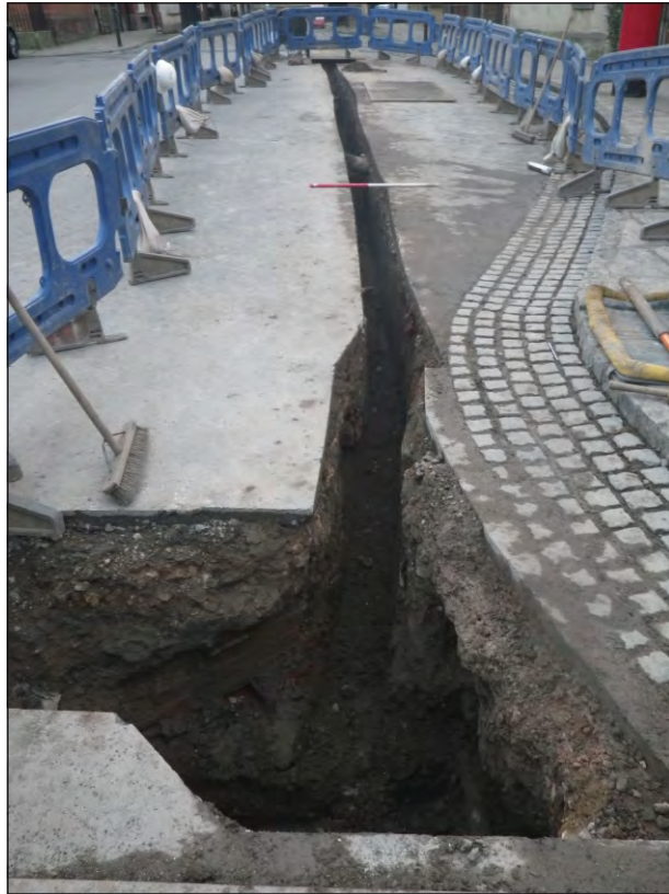
Plate 5: Trench 19 in Heritage Zone 1, camera facing south-west
