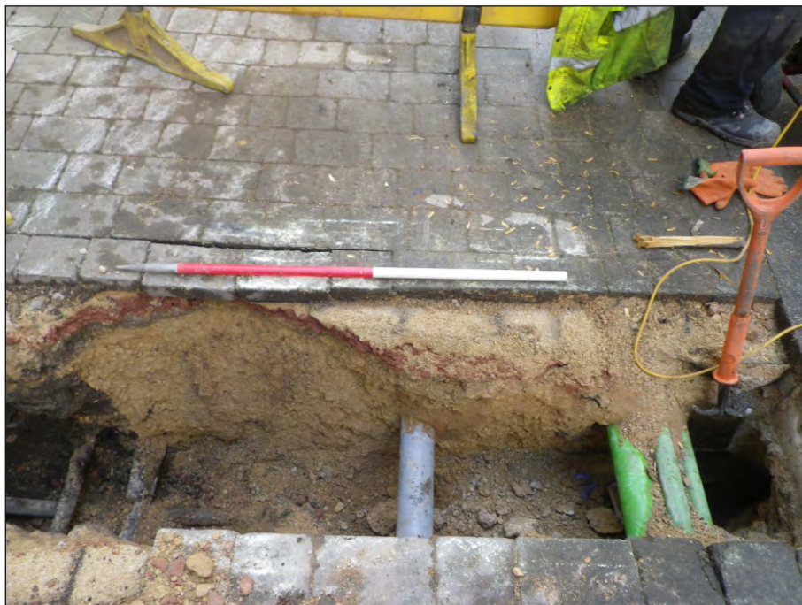
Plate 26: Trench 84 in Heritage Zone 9, camera facing south-west
