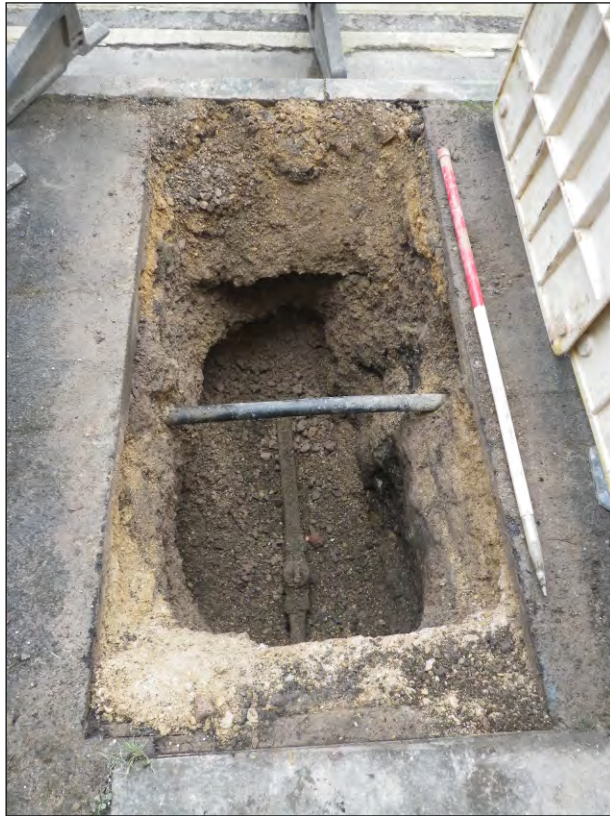
Plate 17: Trench 35 in Heritage Zone 5, camera facing north-east
