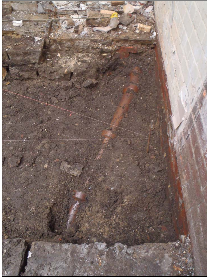
Plate 5: Sewer 1002/1003 looking east
