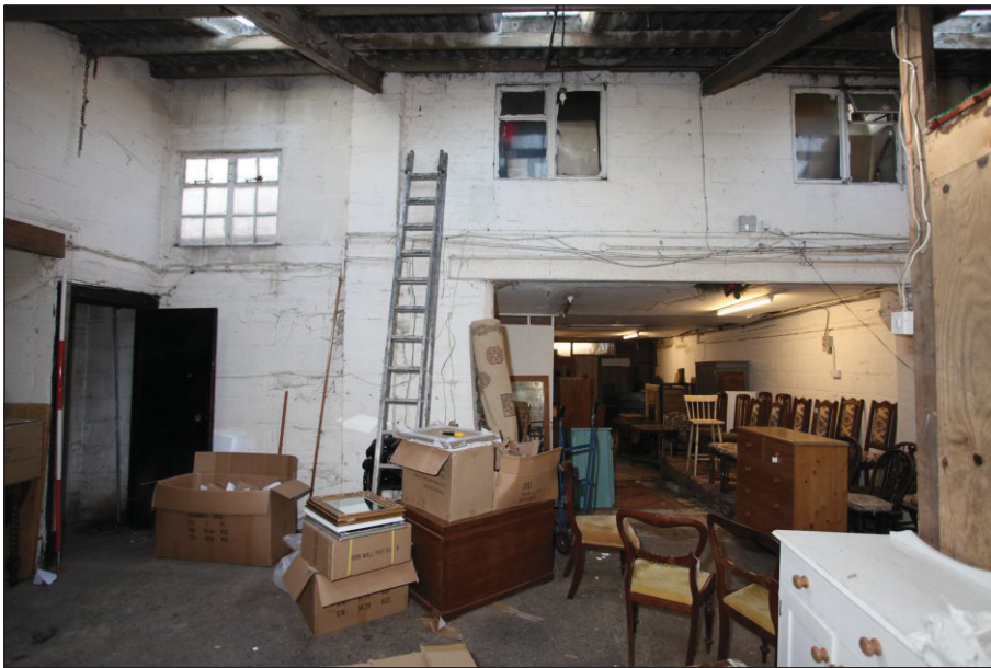
Plate 8: South-facing view of the internal elevation of the south wall of the lean-to
