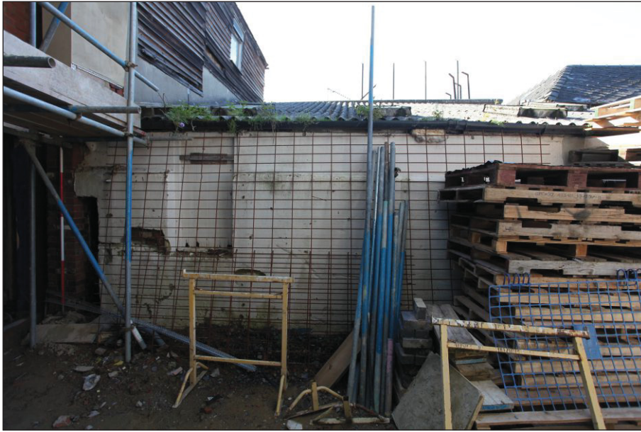
Plate 7: External elevation of the lean-to showing the blocked window
