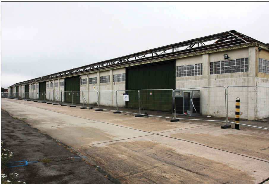
Plate 4: North-west elevation of Building 1
