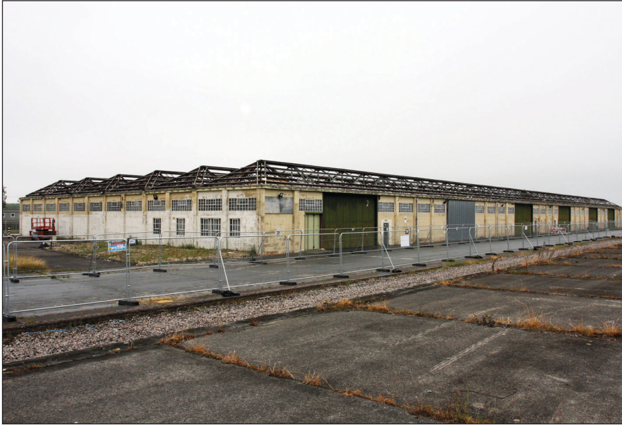
Plate 3: Oblique view of the south-west and south-east elevations of Building 1
