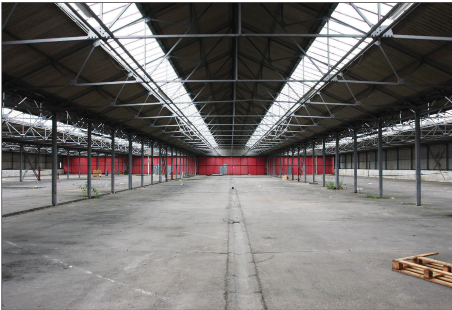
Plate 16: View from the south-east of the interior of Building 105
