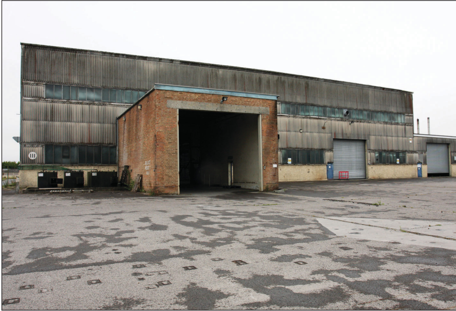
Plate 9: North-west elevation of Building 111
