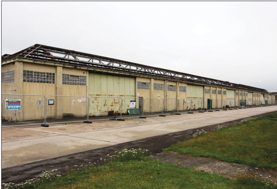
Plate 7: North-west elevation of Building 2
