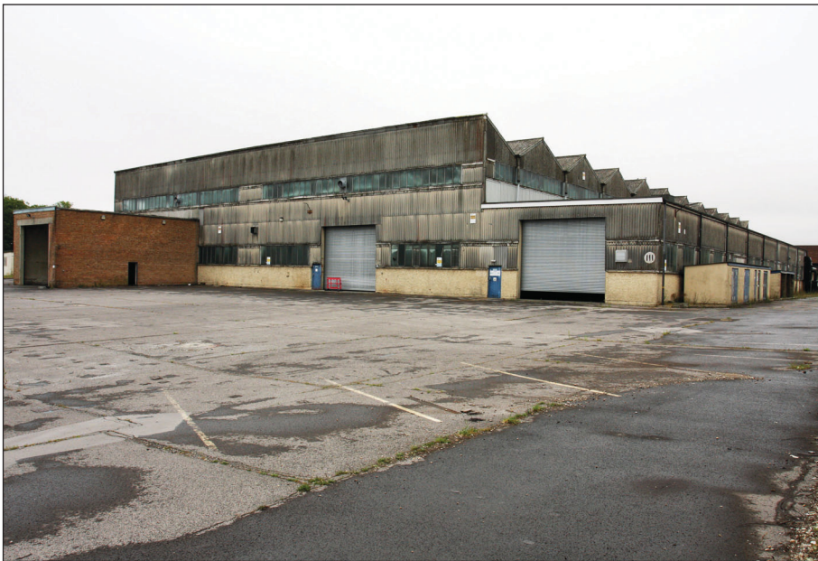
Plate 10: Oblique view of the north-west and south-west elevations of Building 111
