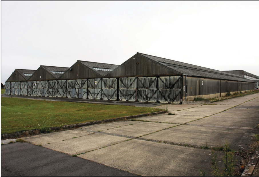
Plate 15: Oblique view of the north-west and south-west elevations of Building 105
