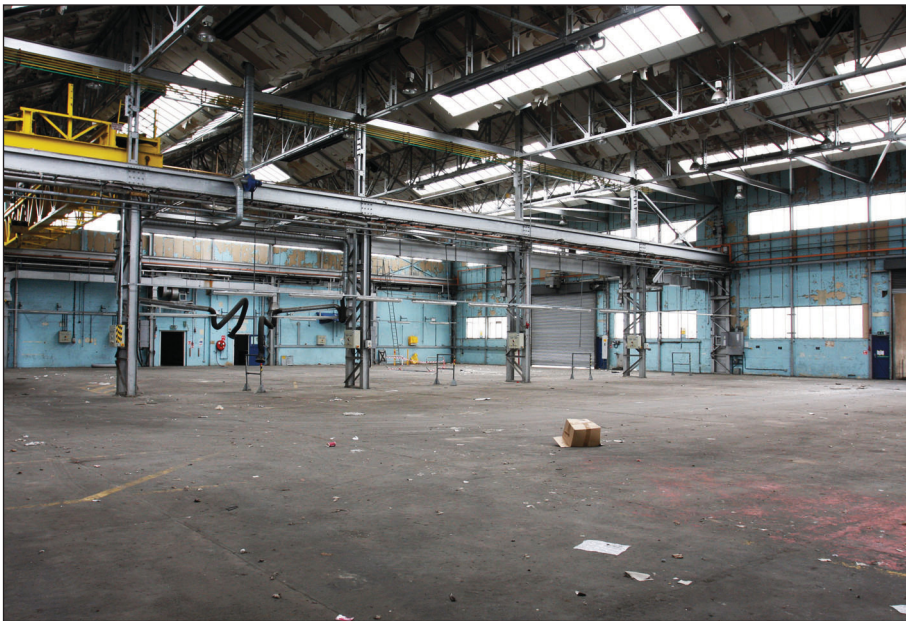
Plate 12: View from the east of the southern workshop of Building 111.
