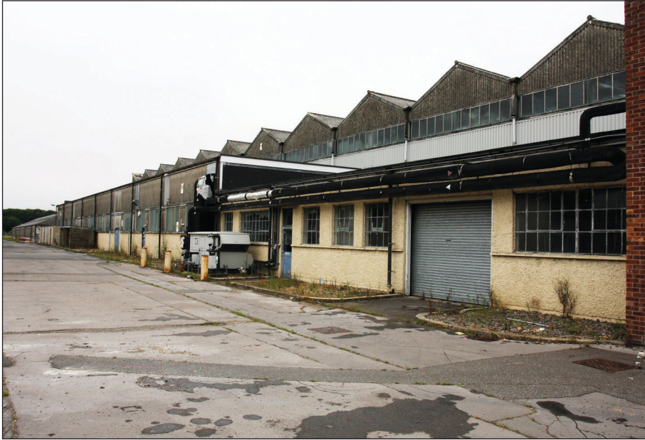
Plate 11: South-west elevation of Building 111.
