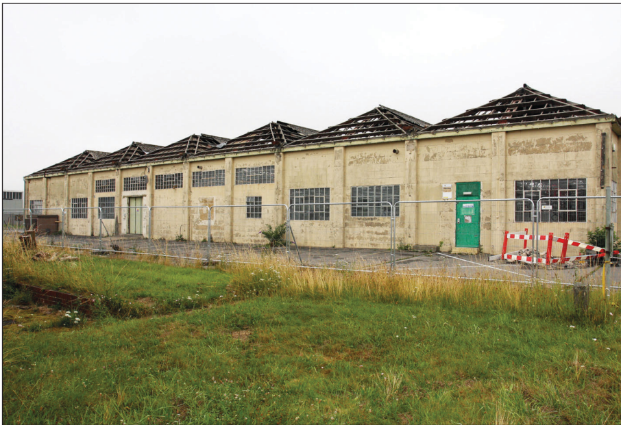
Plate 6: South-west elevation of Building 2
