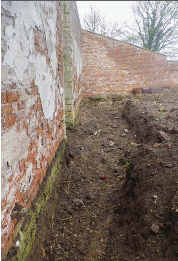
Plate 9: Trench 4, adjacent to the garden wall, facing the north-east corner
