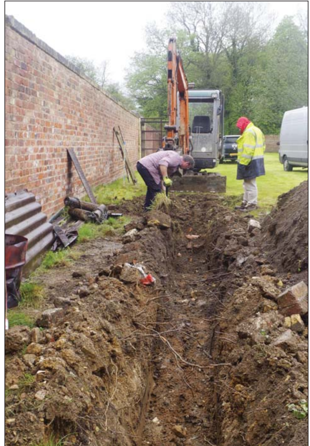
Plate 10: Trench 4, showing the excavation of the north-south pipe trench
