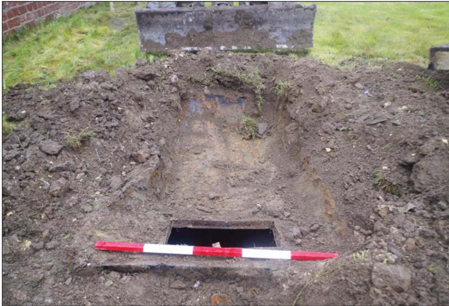
Plate 11: Trench 4, the re-discovered steel soak-away tank
