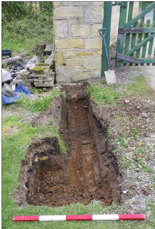
Plate 4: Trench 1, showing the stone pier due to be re-sited
