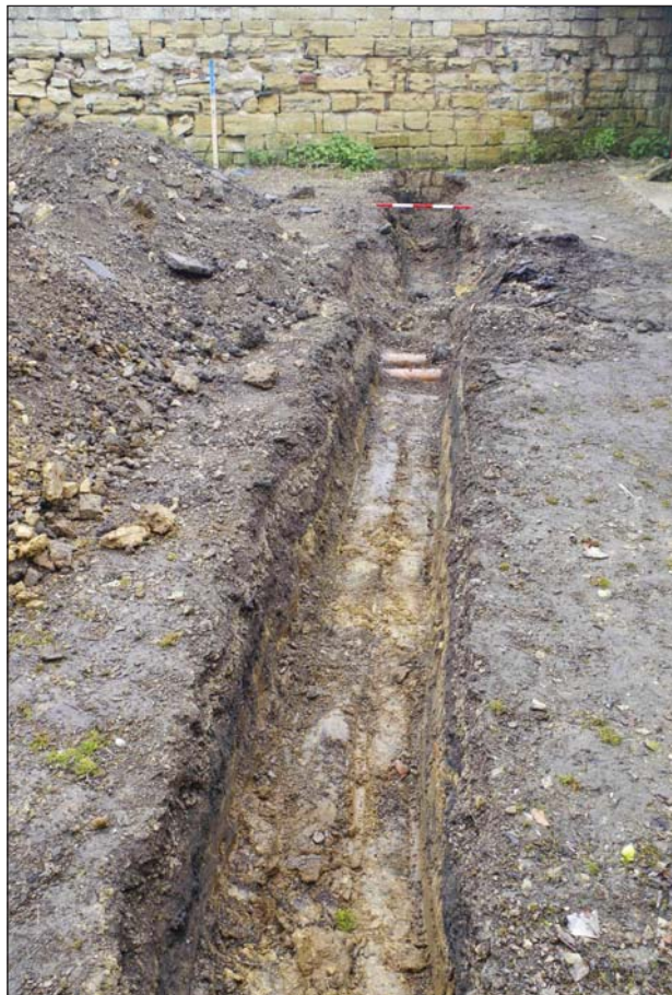
Plate 6: Trench 3, foundation trench extending to the eastern boundary wall
