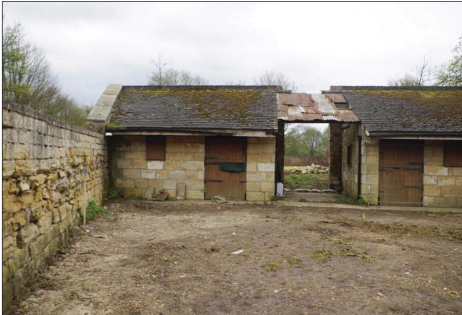
Plate 2: Late 20th century stables facing an open yard
