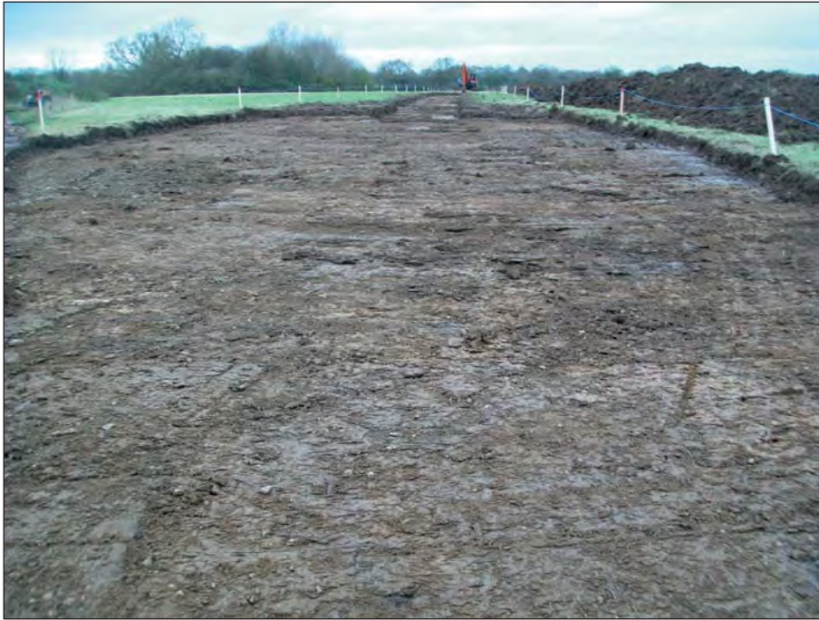
Plate 3: Topsoil strip for open cut excavation
