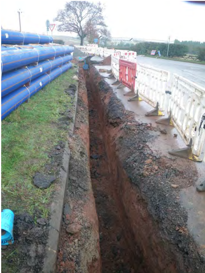
Plate 1: Trenching to south of crossroads
