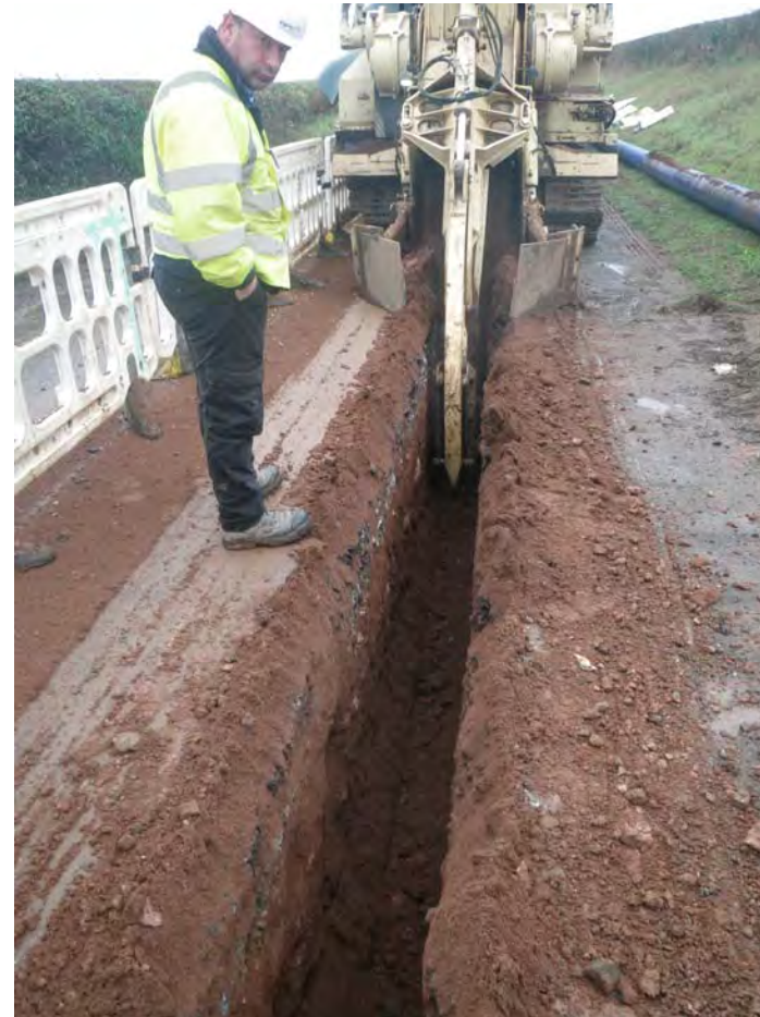
Plate 2: Trench cutter continuing South
