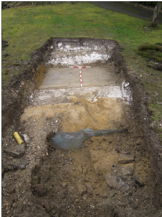
Plate 4: Trench 2 from the east showing blue fibreglass lining of swimming pool (scale 1m, 0.50m)
