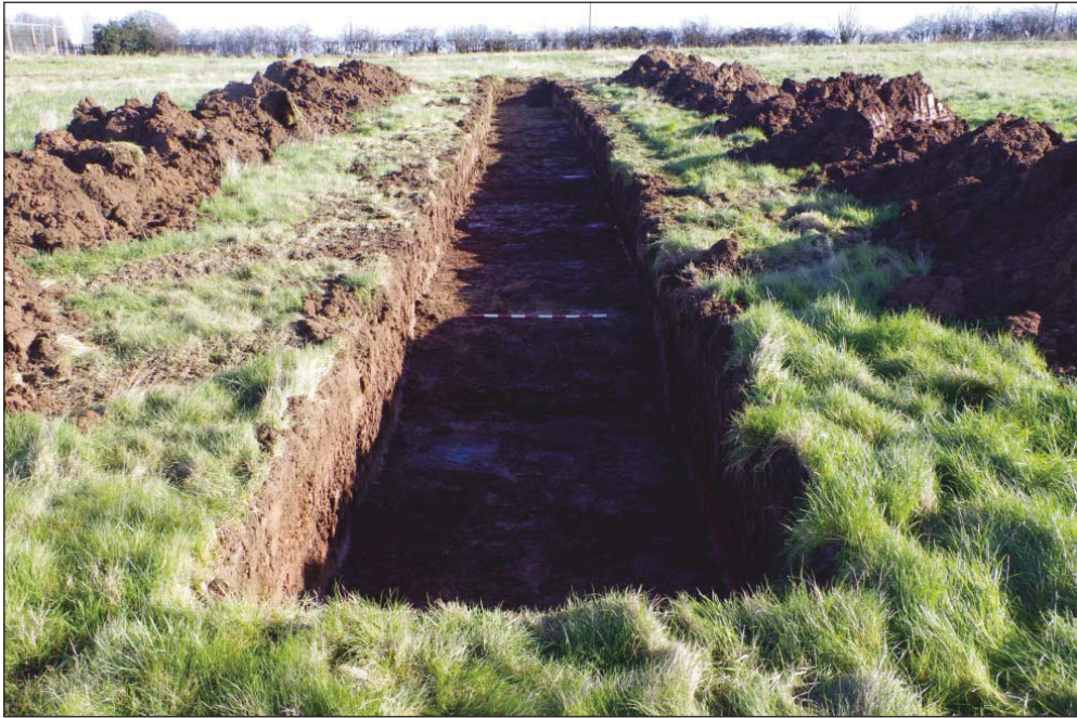
Plate 1: General shot of Trench 1, facing north-east
