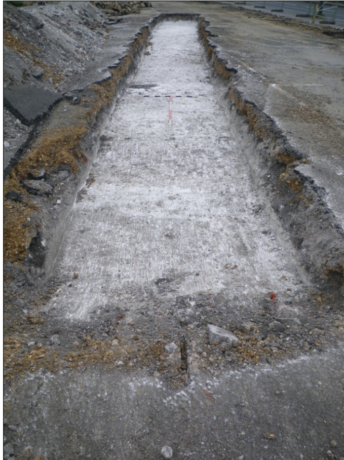
Plate 5: Trench 3, view from north
