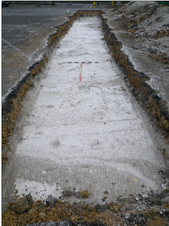
Plate 1: Trench 1, view from west
