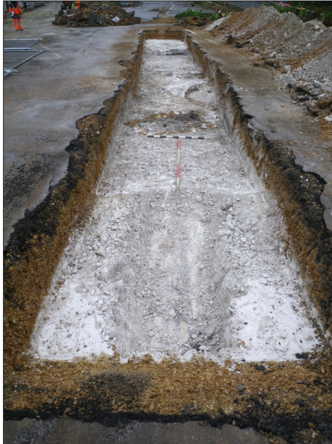
Plate 7: Trench 4, view from south
