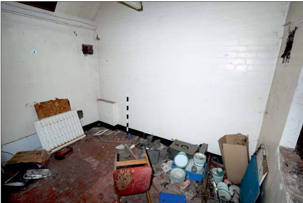
Plate 18: Interior of pre WW1 kitchen extension
