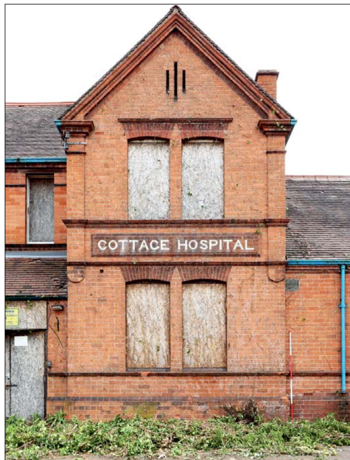
Plate 2: Two storey projection showing architectural detailing
