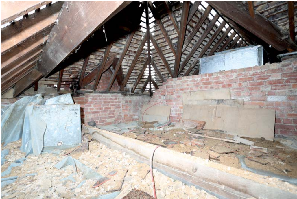
Plate 16: Interior of main roof
