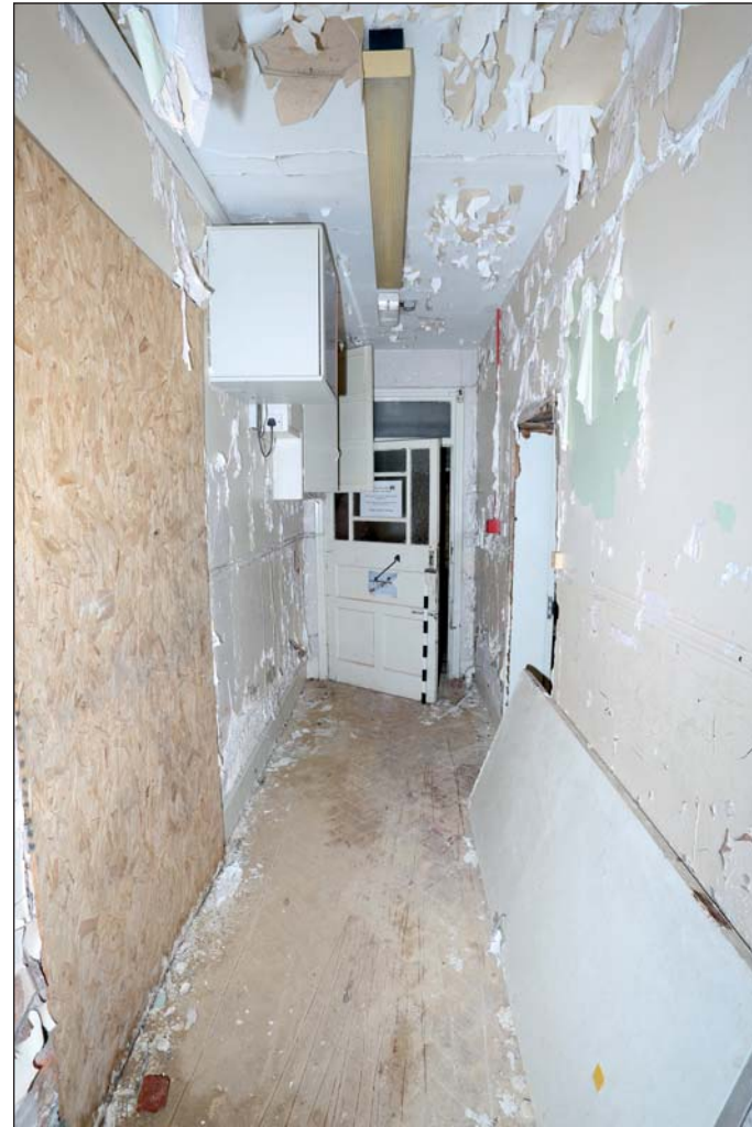
Plate 10: Main entrance with original door
