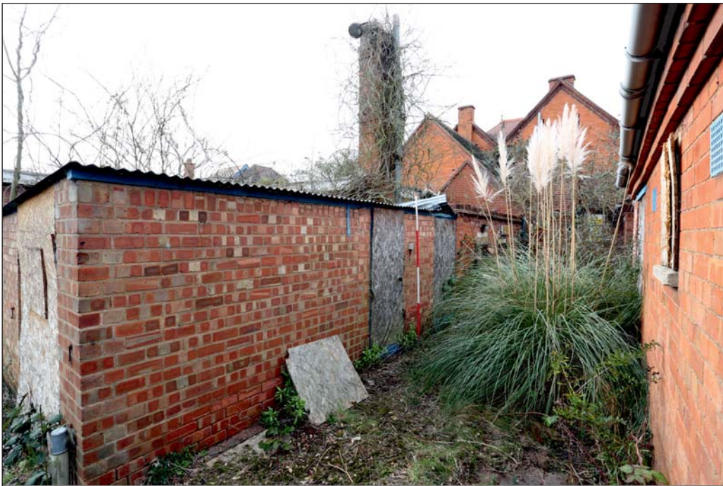
Plate 22: View of boiler house and chimney, behind pampas grass
