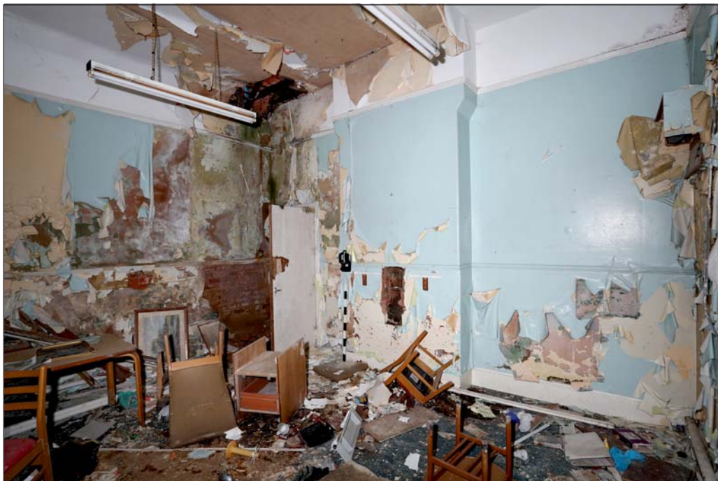
Plate 6: Staff dining room showing original dado, picture rail, skirting and chimney
