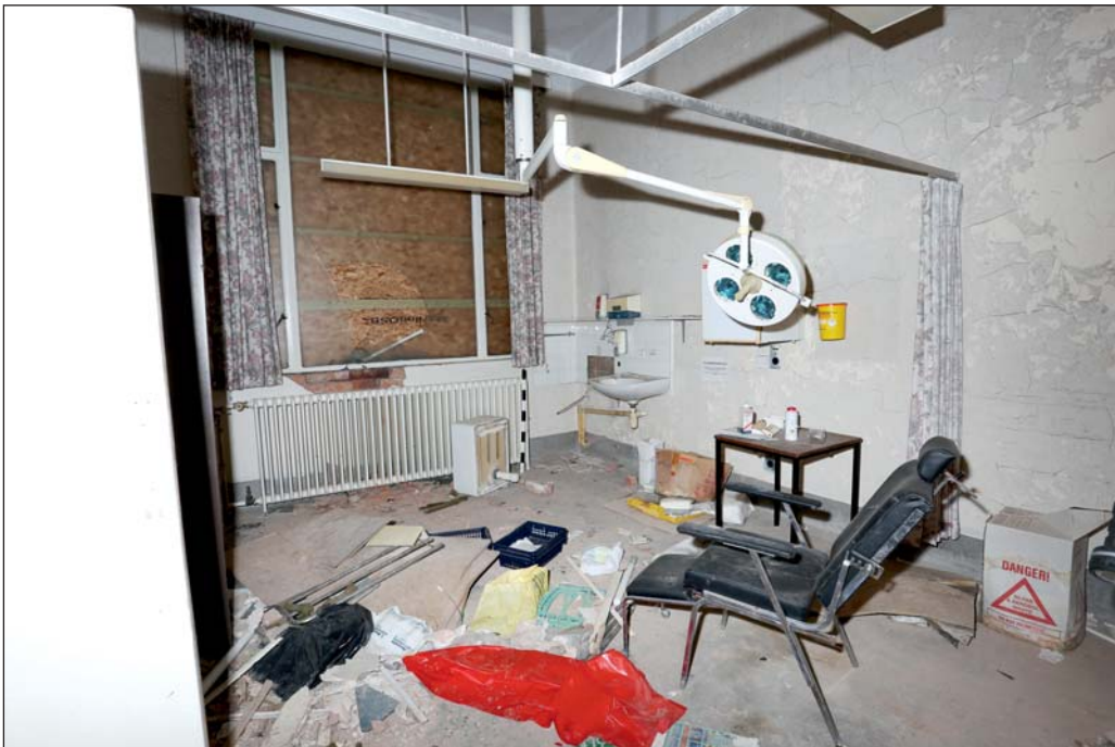
Plate 24: 1937 operating theatre showing original window
