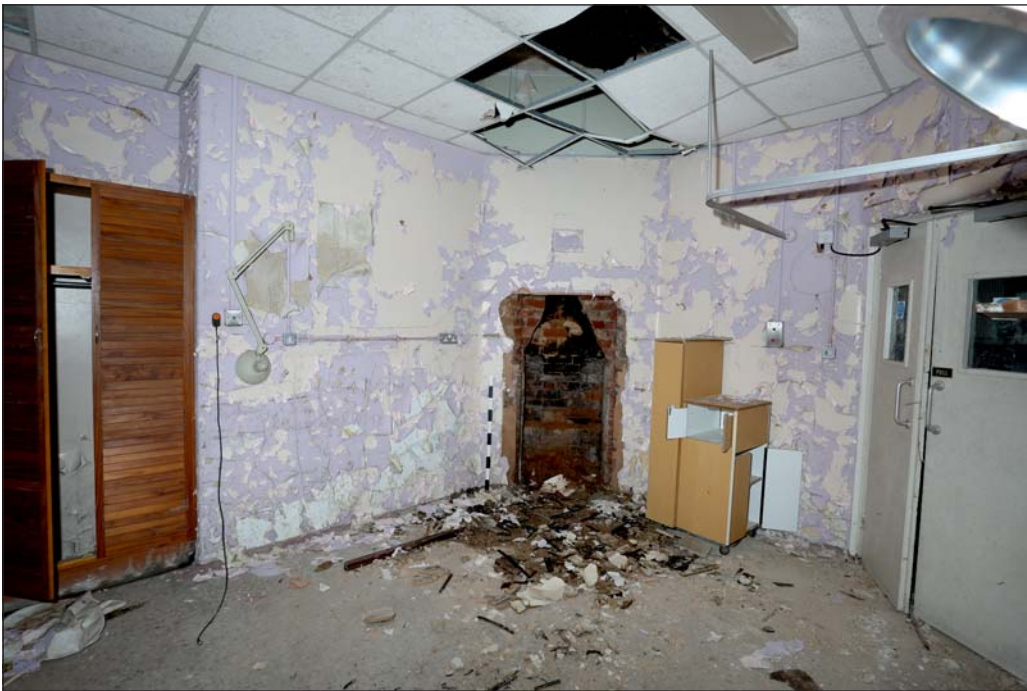
Plate 12: Altered original ground floor room
