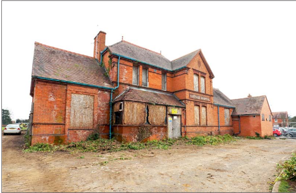
Plate 1: West front viewed from north-west
