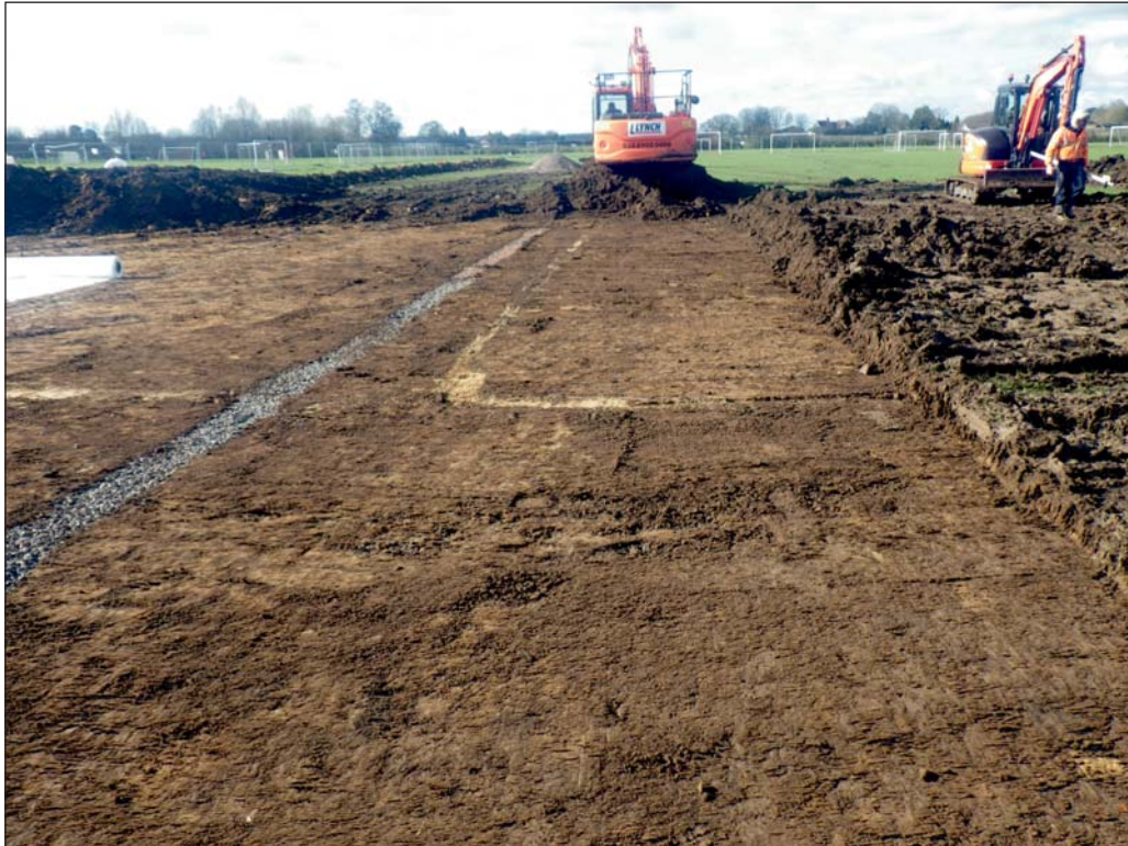
Plate 5: Topsoil stripping of proposed sports pitch taken from the east
