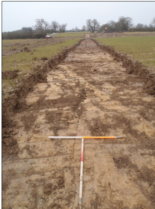
Plate 5: General view of Access Road 3, facing south
