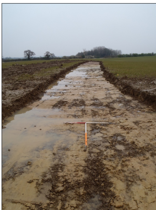
Plate 1: General view of Access Road 1, facing south
