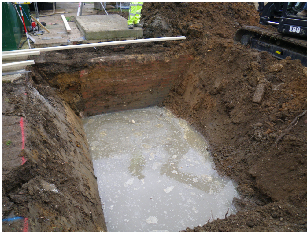
Plate 2: Trench 1 with red brick wall [105]
