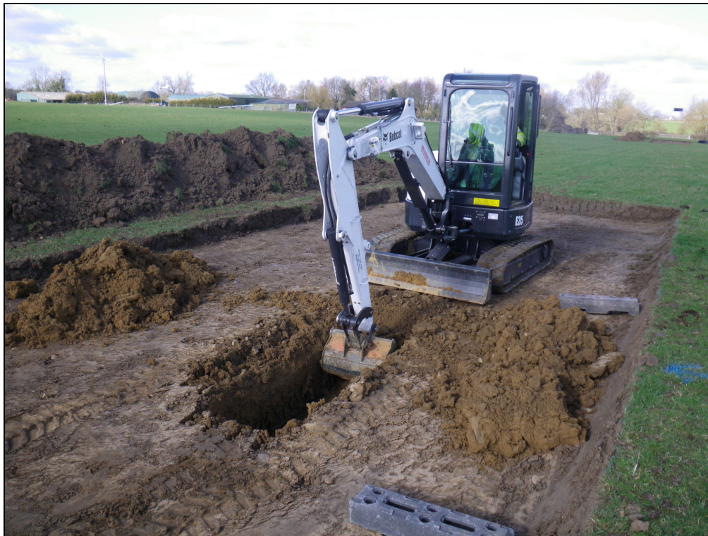
Plate 1: Trench 11 including stripped area, view from south
