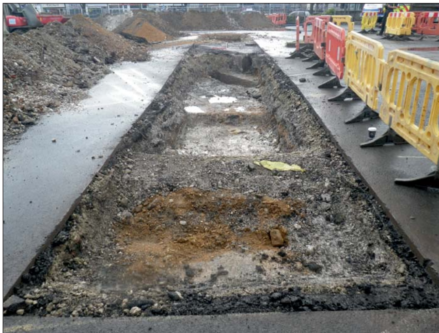
Plate 8: Trench 11, concrete footings, view from north west
