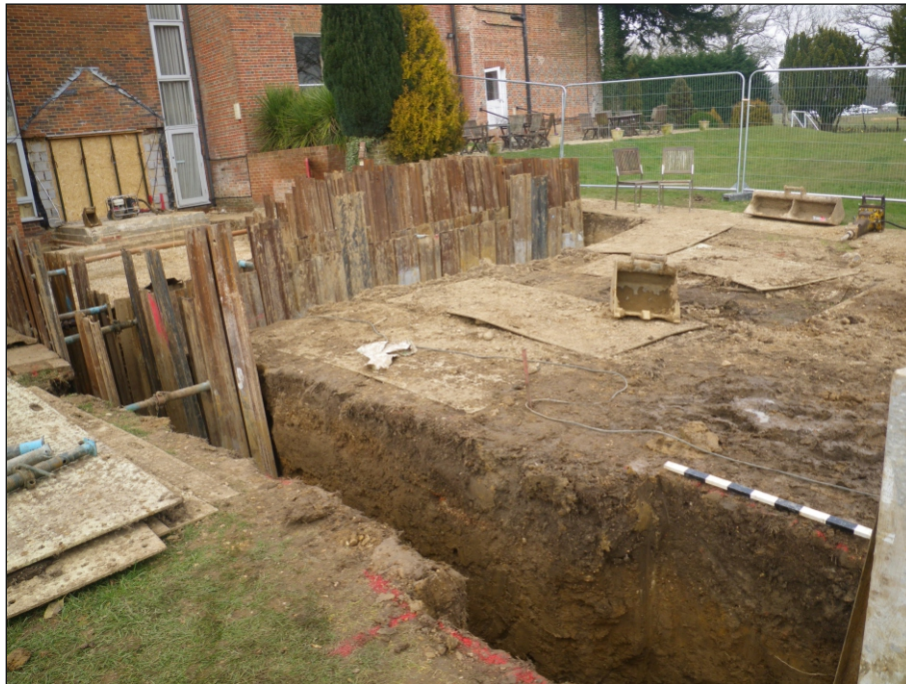
Plate 5: Retention wall trench with section (TR 2), view from south-west
