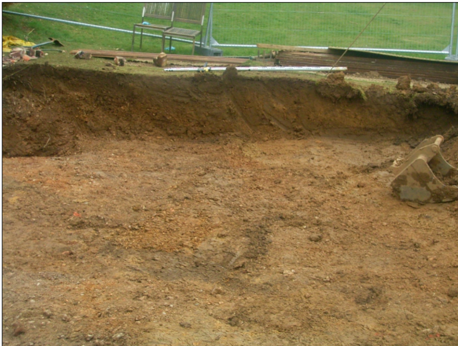
Plate 2: Restaurant extension strip area with section, view from south-west
