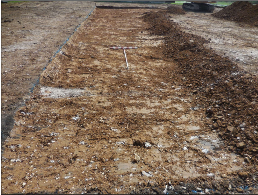
Plate 1: Reduced dig for building viewed from the west
