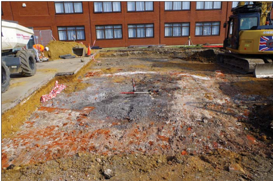
Plate 4: Structures 310, 331 and 332, viewed from the north-west
