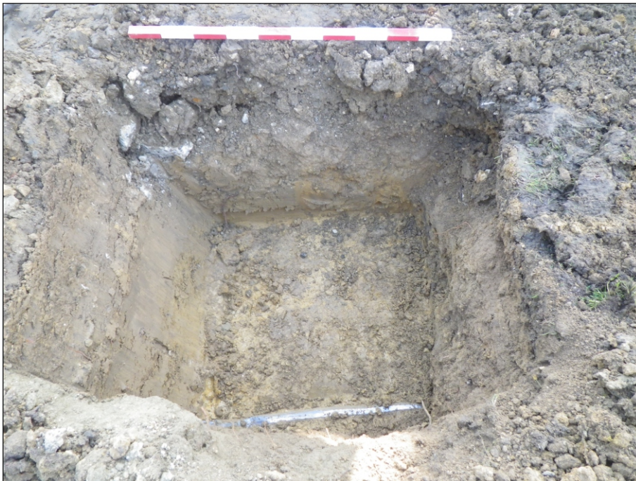
Plate 4: West facing section of footing for Pad 65
