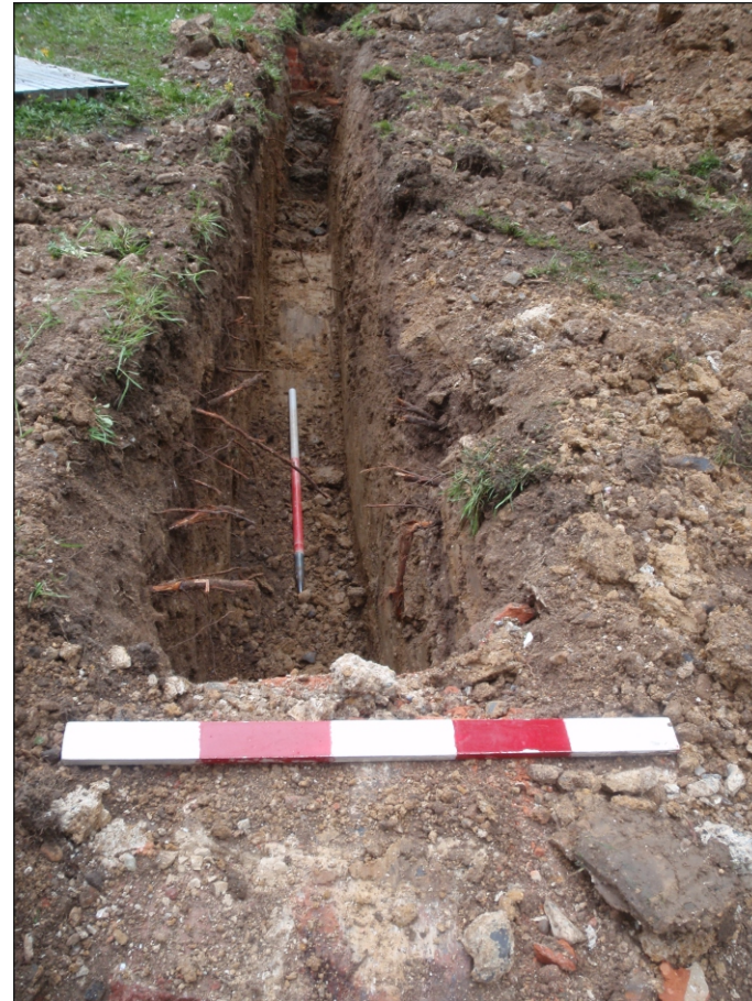
Plate 6: Modern wall in pipe trench
