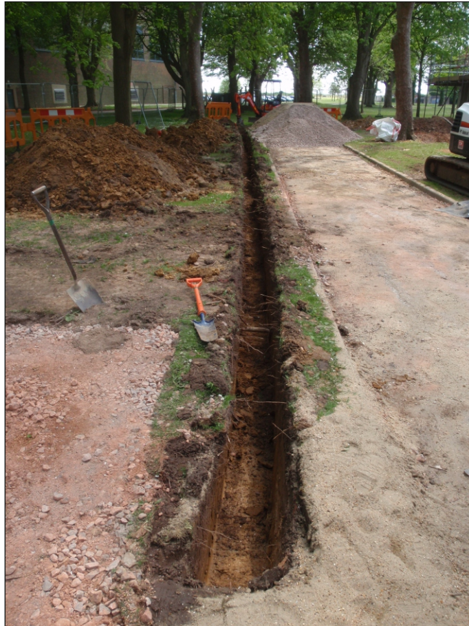
Plate 5: Pipe trench from the north
