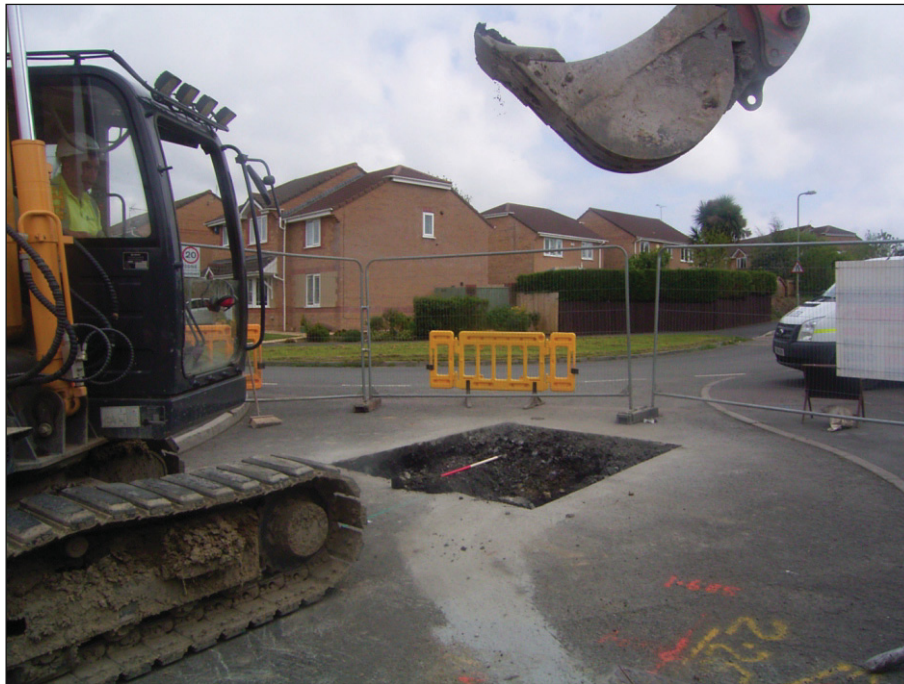
Plate 9: Test pit 1 from the north-west
