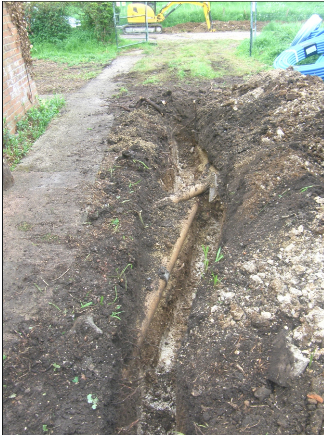
Plate 3: Ducting trench by cottages at the north-western end of the Route
