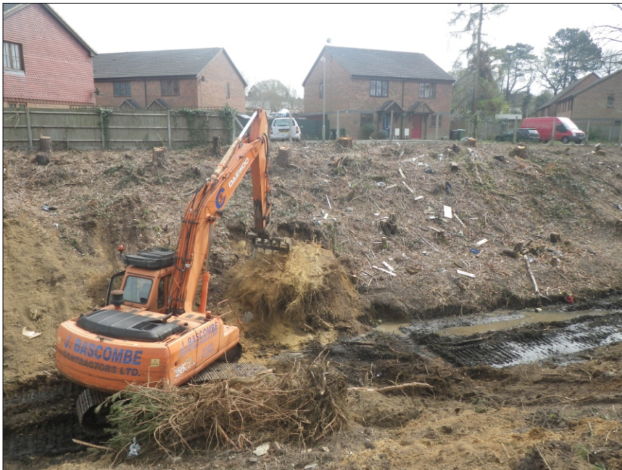
Plate 6: Stump removal using an excavator fitted with a rake attachment
