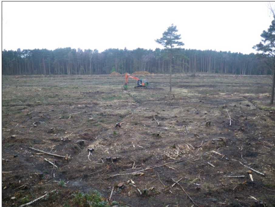
Plate 1: View of the northern part of the watching brief area
