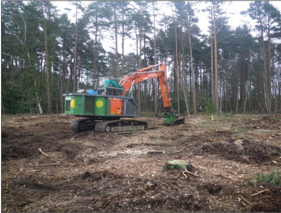
Plate 5: Stump removal with an excavator fitted with a grinder
