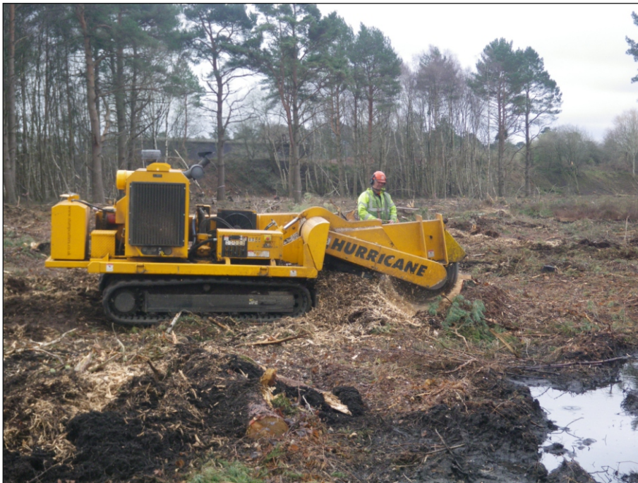
Plate 4: Stump removal process using a stump cutter
