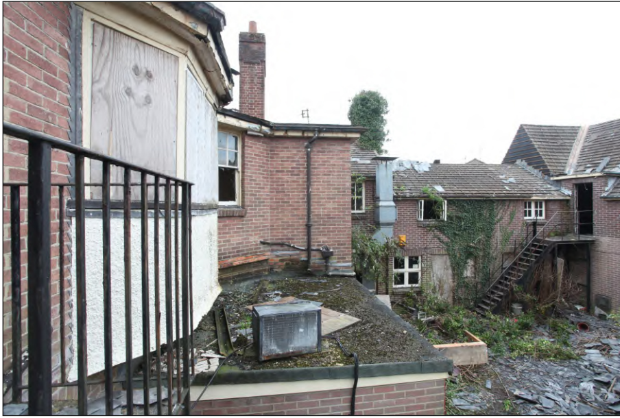
Plate 17: West range of Hotel, looking west
