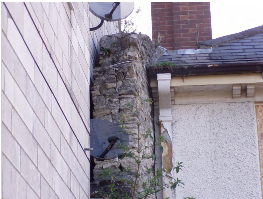
Plate 8: Stub of west gable wall, looking north
