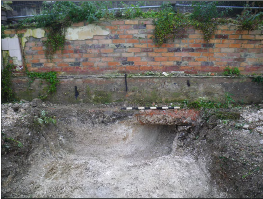
Plate 5: West end of Trench 4, looking west
