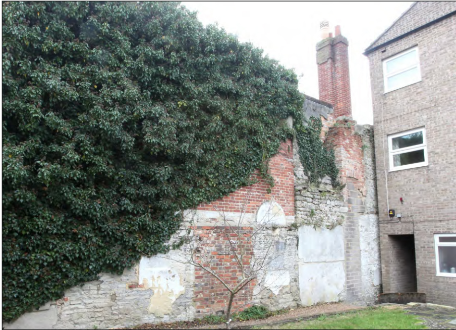
Plate 9: West boundary wall, looking south-east
