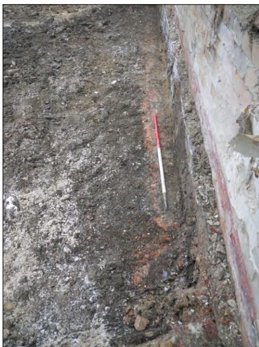
Plate 1: Brick footings by west boundary wall, looking south
