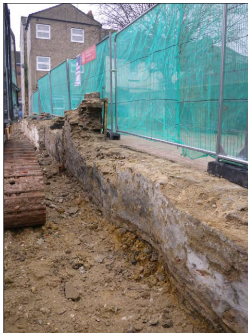
Plate 4: North end of west range with stone wall, looking south-west
