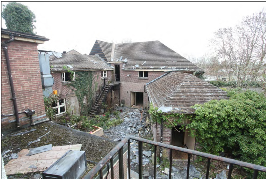
Plate 18: West, north and east ranges, looking north-west
