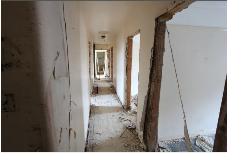
Plate 15: First floor corridor, looking east
