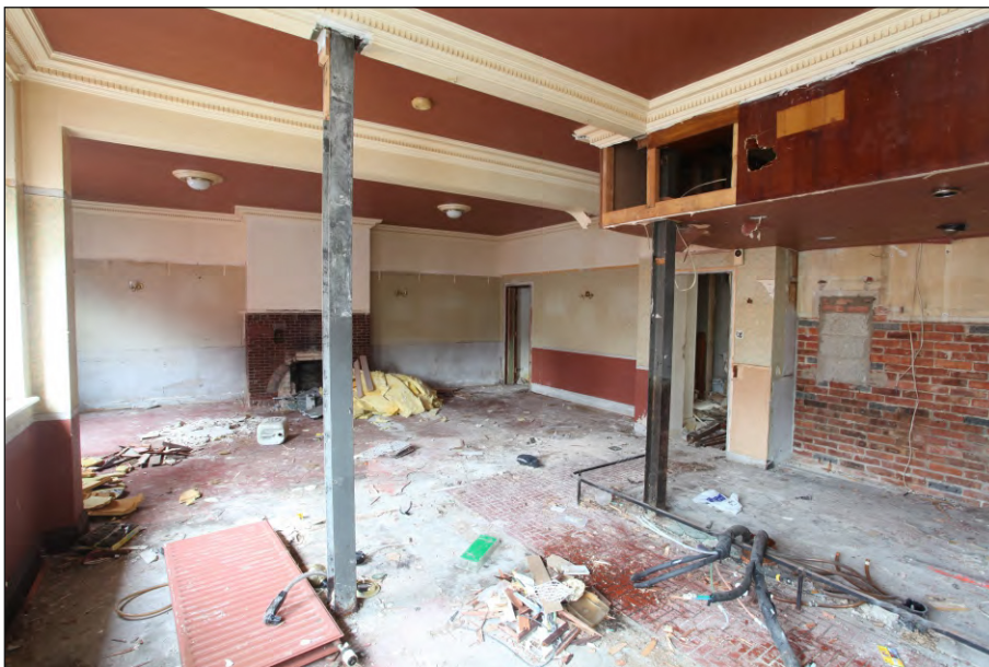
Plate 14: Gentlemen's Bar, looking north-east
