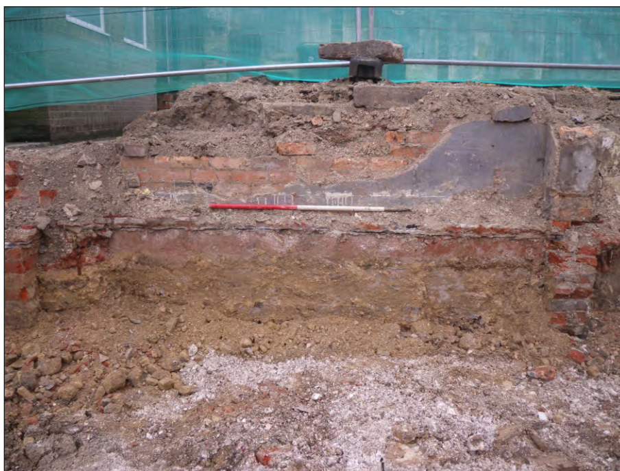
Plate 2: Part of kitchen wall and two partition wall stubs, built up against western stone boundary wall, looking west
