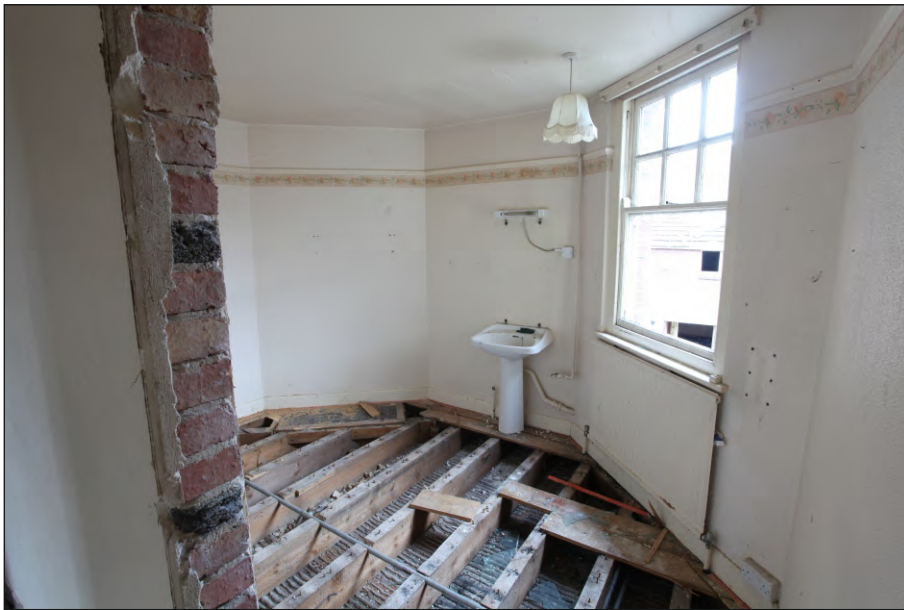
Plate 16: Front bedroom, looking south-east
