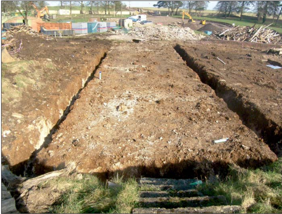
Plate 1: Site shot of part of Trench 2 excavated
