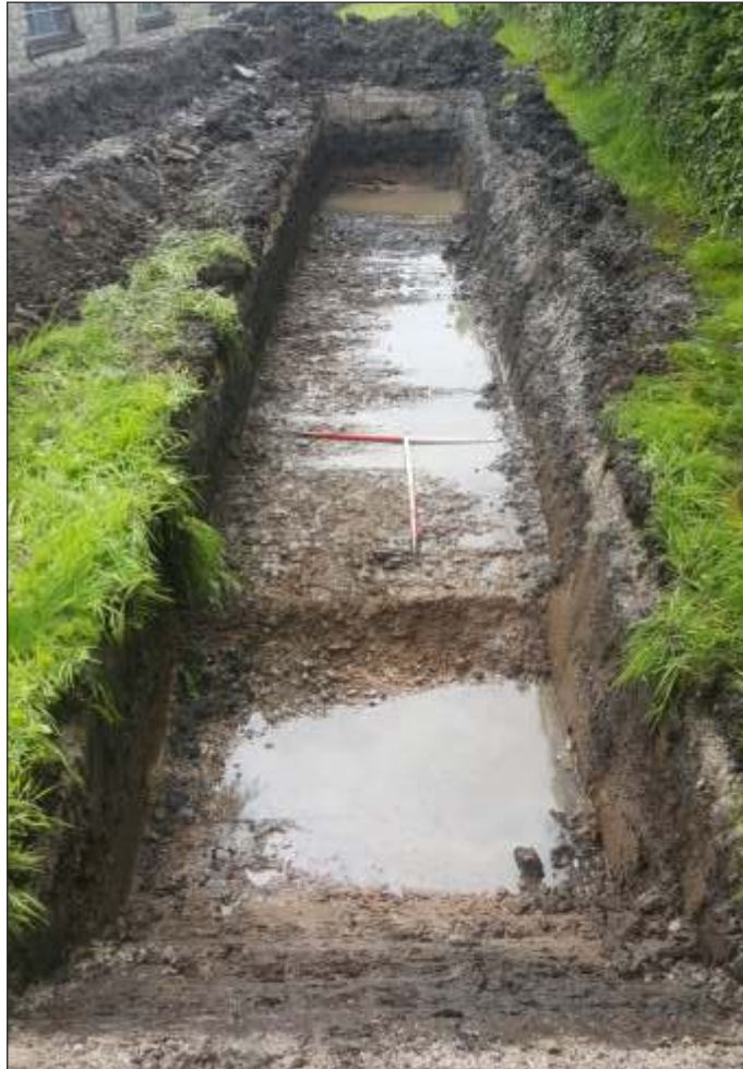
Plate 1: Trench 1, view from north
