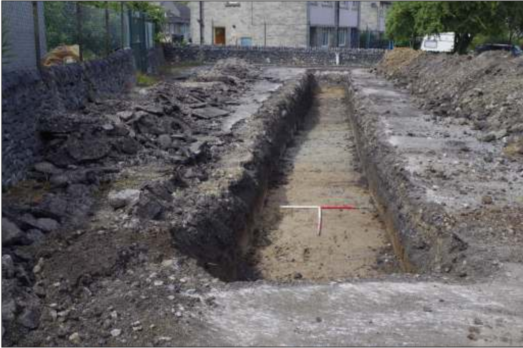
Plate 3: Trench 2, view from south
