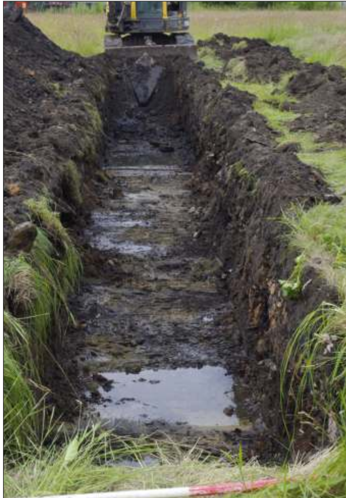
Plate 6: Trench 6, view from south
