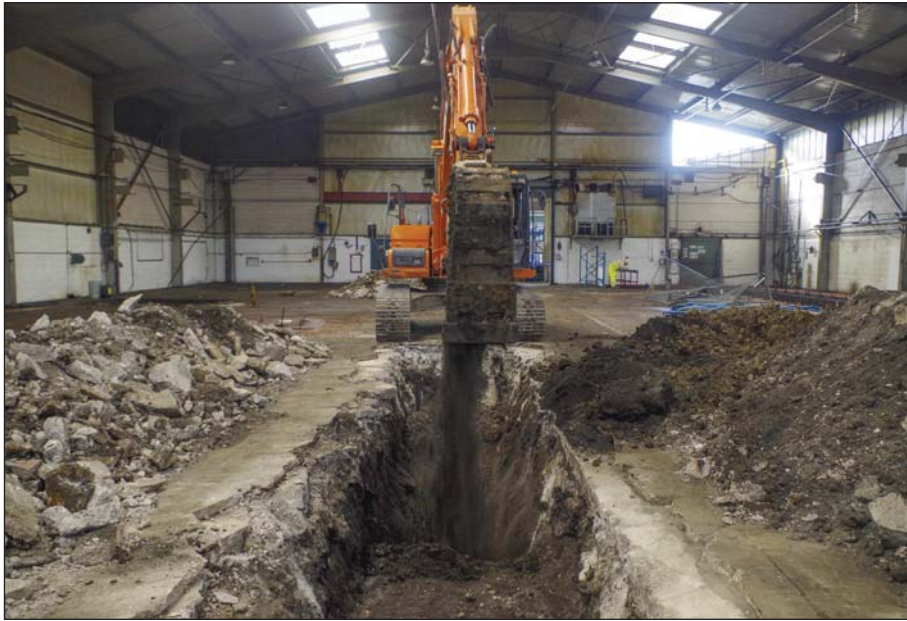
Plate 5: Backfilling 'industrial' deposits into trench 21, looking south
