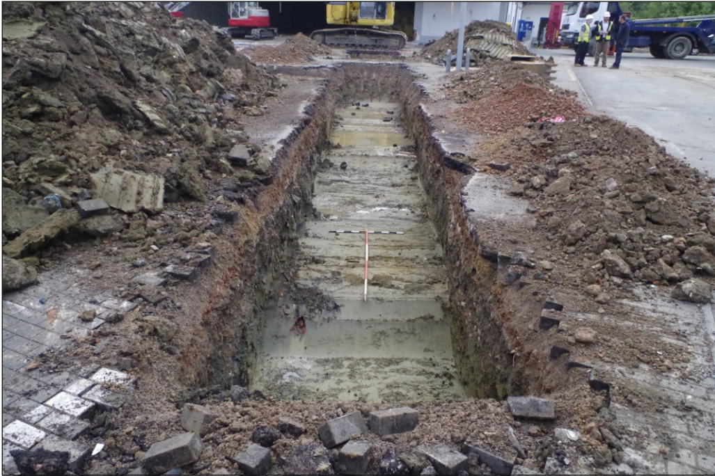
Plate 3: View from the west of Trench 2
