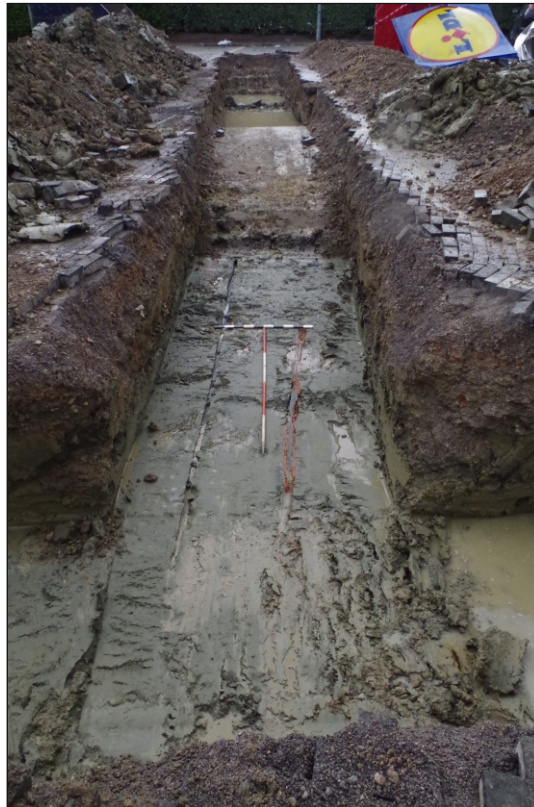
Plate 4: View from the SSW of Trench 2
