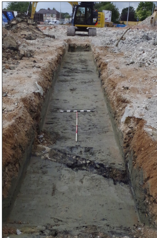
Plate 6: View from the east of Trench 3
