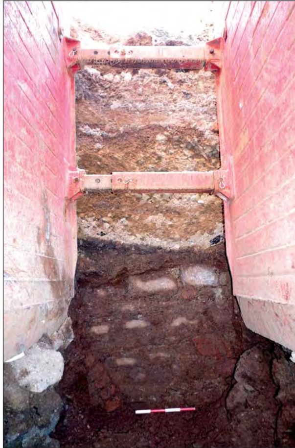
Plate 1: South-west facing elevation of exposed goods shed wall
