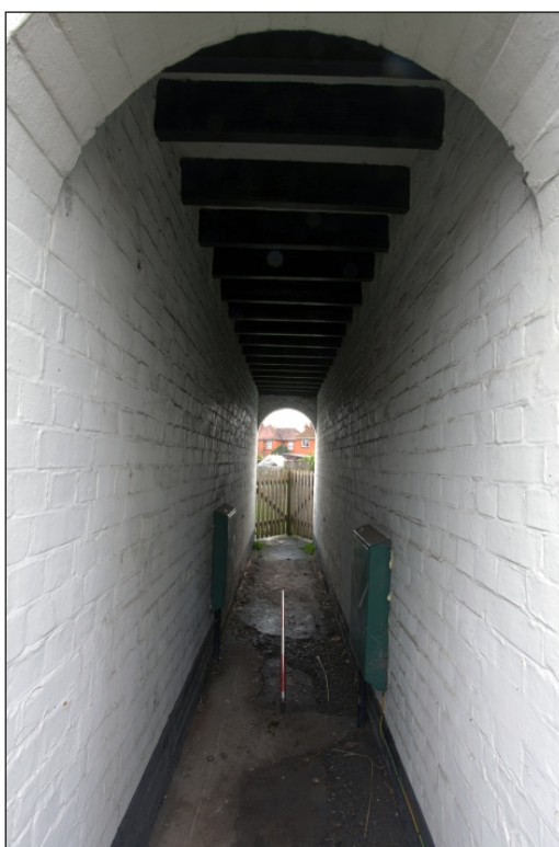
Plate 5: View from the north-west of the arched passage
