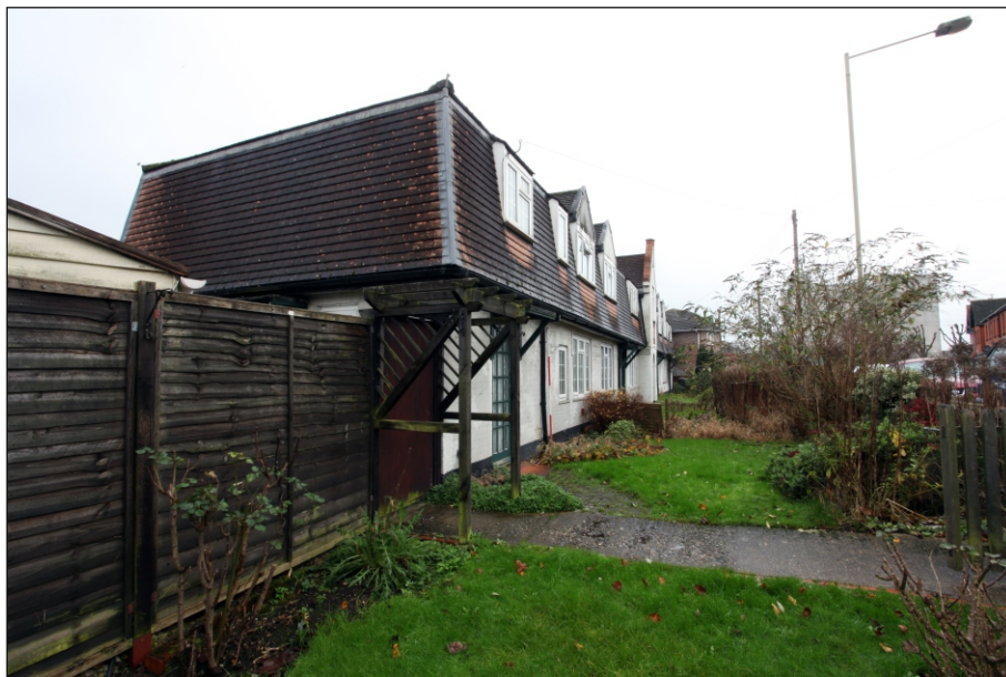
Plate 2: Oblique view of the north-west and north-east elevations showing the front gardens and approach to No. 17 Mill Lane
