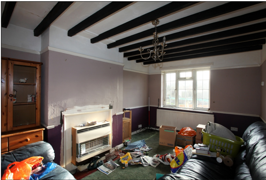
Plate 14: West facing view of the living room and under-stairs cupboard of No. 11
