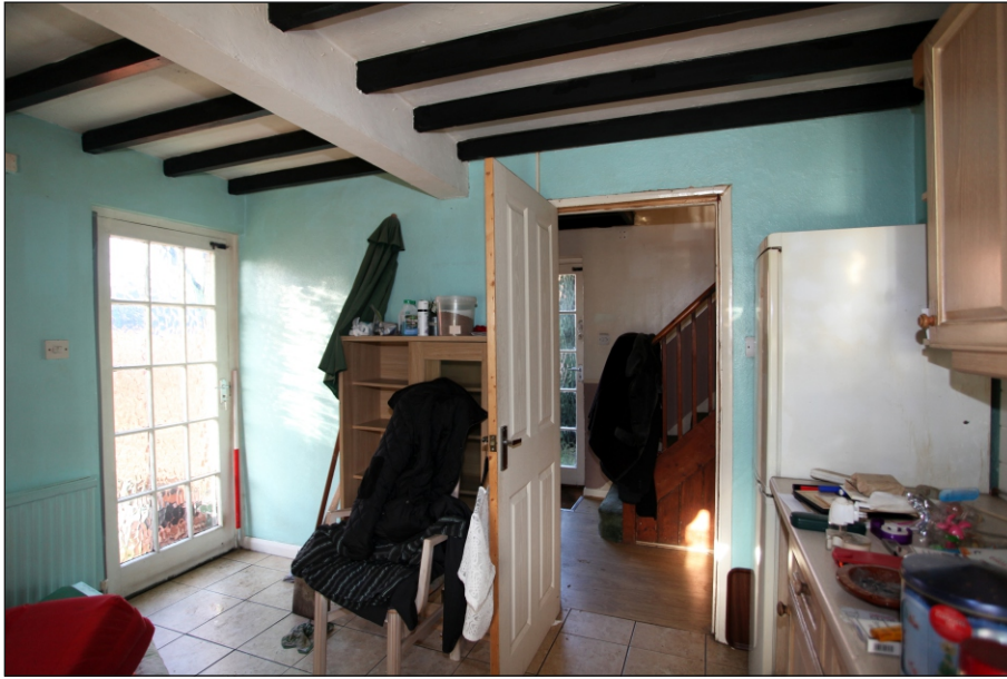
Plate 13: West-facing view of the kitchen on the ground floor of No. 11 with ceiling joists supported on a summer beam
