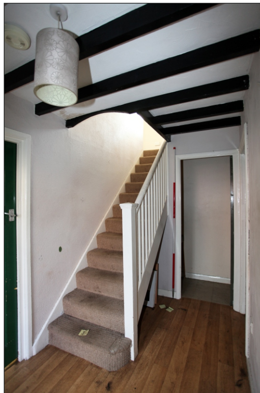
Plate 8: East-facing view of the entrance hall/ stairwell on the ground floor of No. 15
