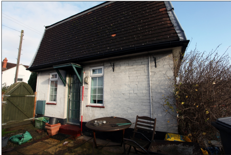
Plate 3: South-west elevation of No. 11 Mill Lane
