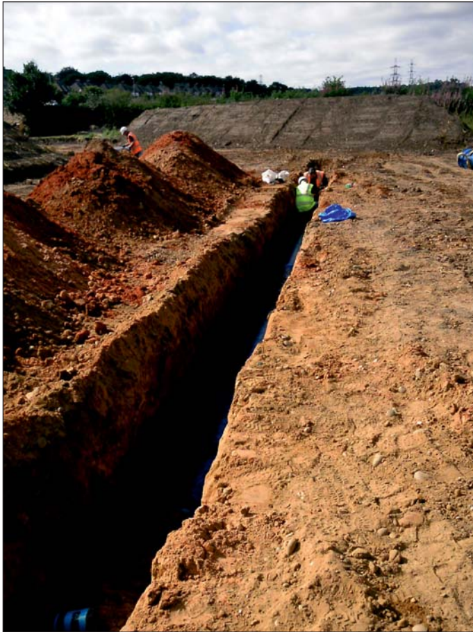
Plate 1: Trench 20, pipe trench
