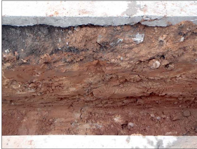
Plate 3: Representative section, Trench 24, George Fredrick Road
