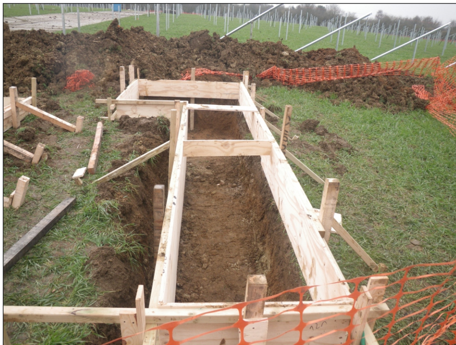
Plate 2: View of excavated trenches for footings of inverter
