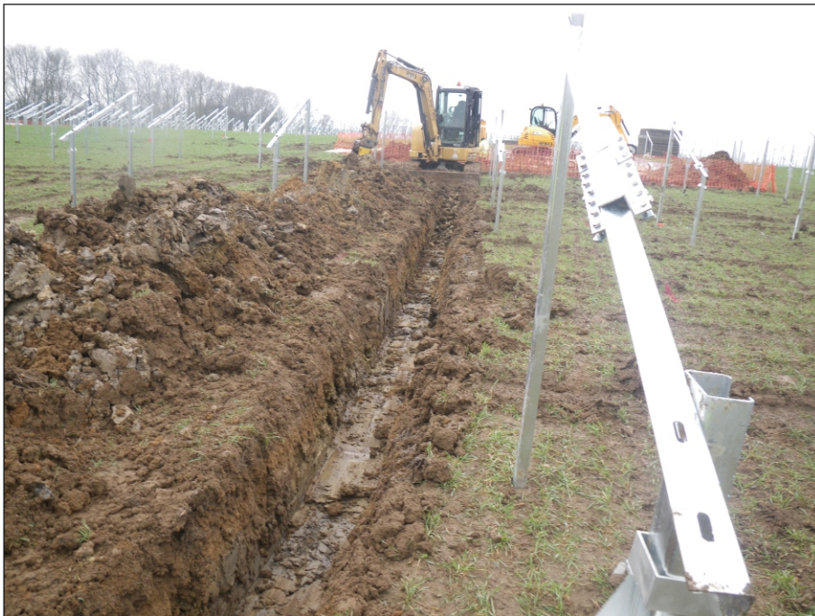
Plate 4: View of excavation of a cable trench
