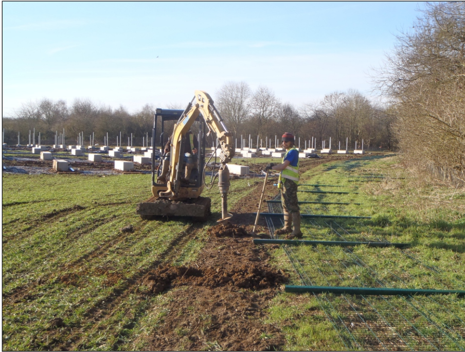
Plate 5: Working shot of boring of holes for perimeter fence
