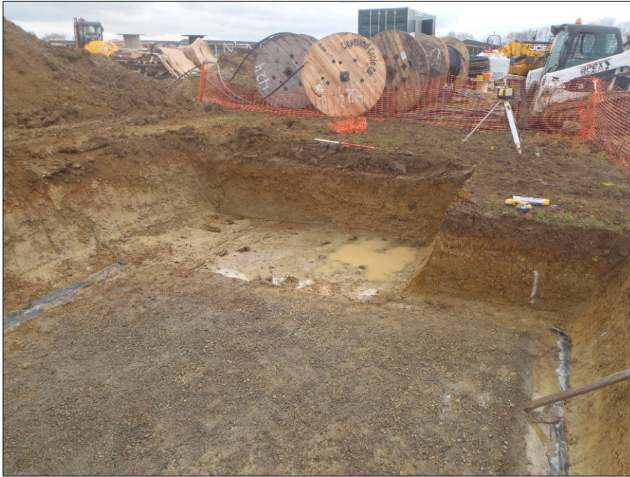
Plate 3: View of excavated area for sub-station
