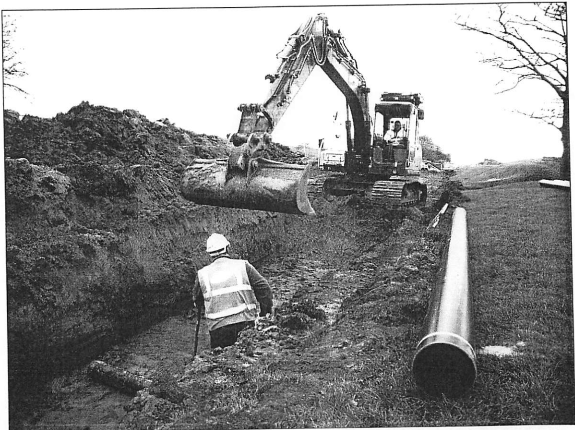
Plate 2: Layer 114 at base of cable trench
