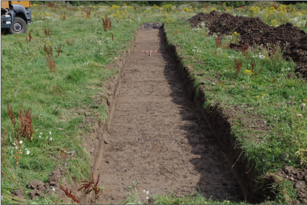
Plate 7: Trench 16, viewed from the southeast
