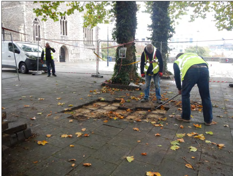
Plate 1: Removing the paving slabs above the area of subsidence, from north-west
