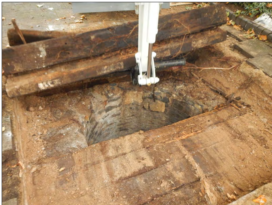
Plate 2: Lifting the timber sleepers covering the well shaft, from north-west
