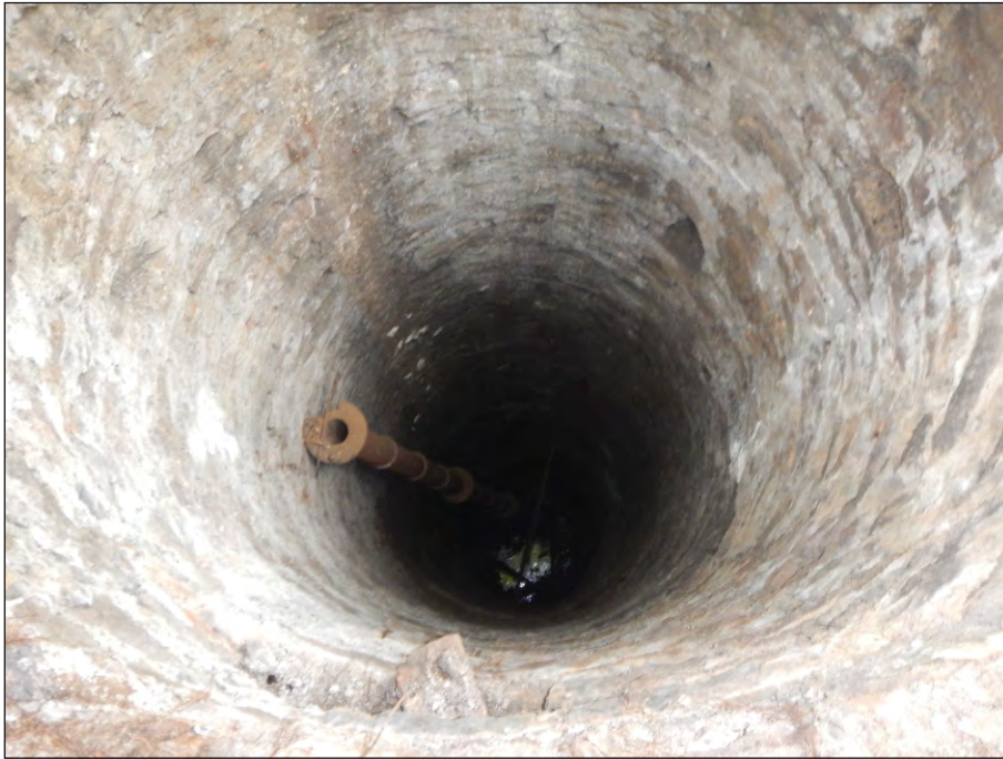
Plate 5: St Edith's well shaft; showing pump pipework, from north
