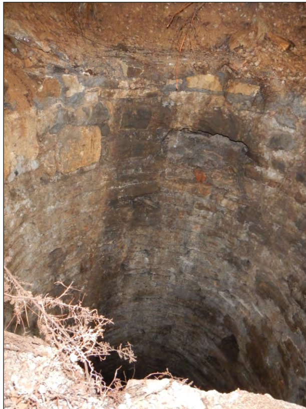
Plate 4: The inner face of the well shaft, from north
