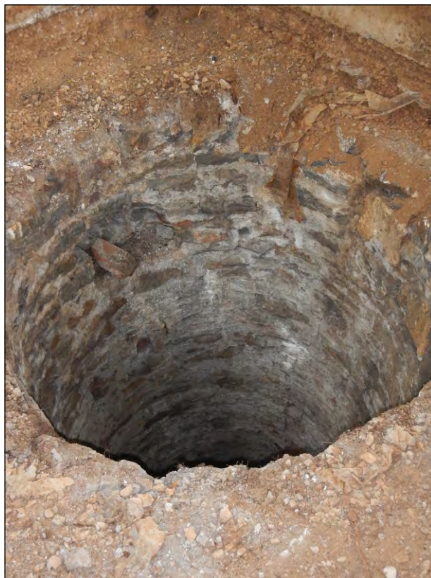
Plate 6: Small openings in the shaft wall, north-east side, from south-west
