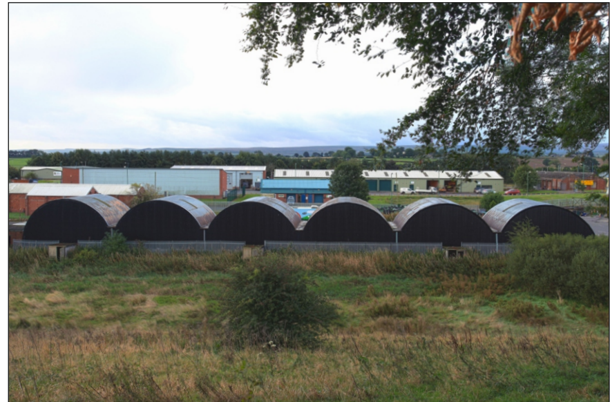
Plate 11: View of the north elevation of the tank garages (Romney sheds)
