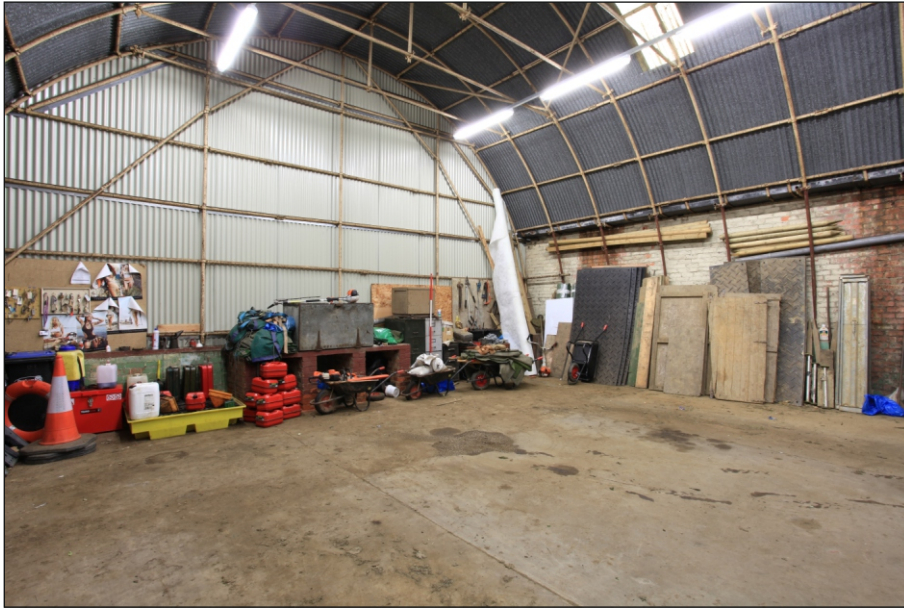
Plate 24: General view of G1, looking north-east
