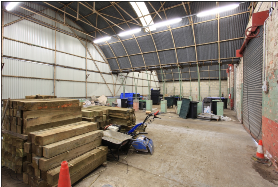
Plate 31: General view of G4 and G5, looking north-east
