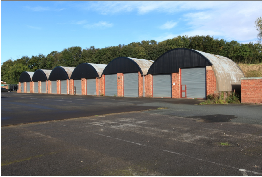
Plate 8: Oblique view of the south elevation of the tank garages (Romney sheds), looking north-west
