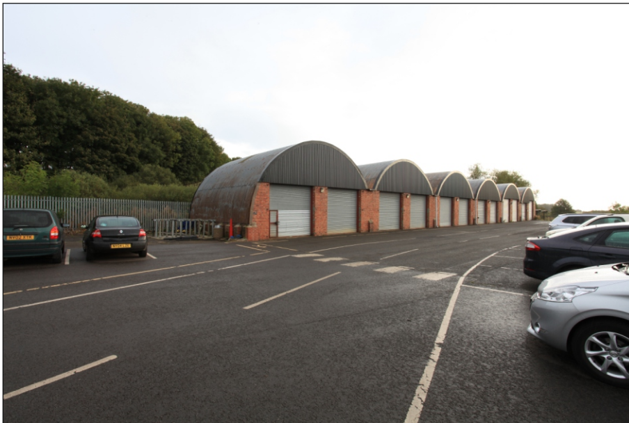
Plate 6: General view of the tank garages (Romney sheds), looking north-east
