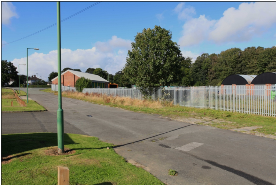
Plate 4: General view of the Site showing the former gatehouse, looking north-west
