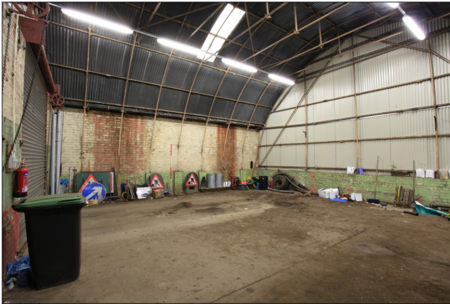
Plate 28: General view of G2, looking north-west
