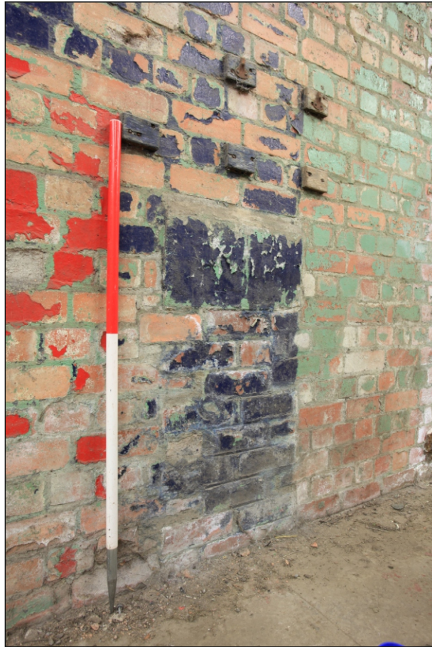
Plate 18: Detail of an embedded pier with the south wall of the tank garages (Romney sheds)
