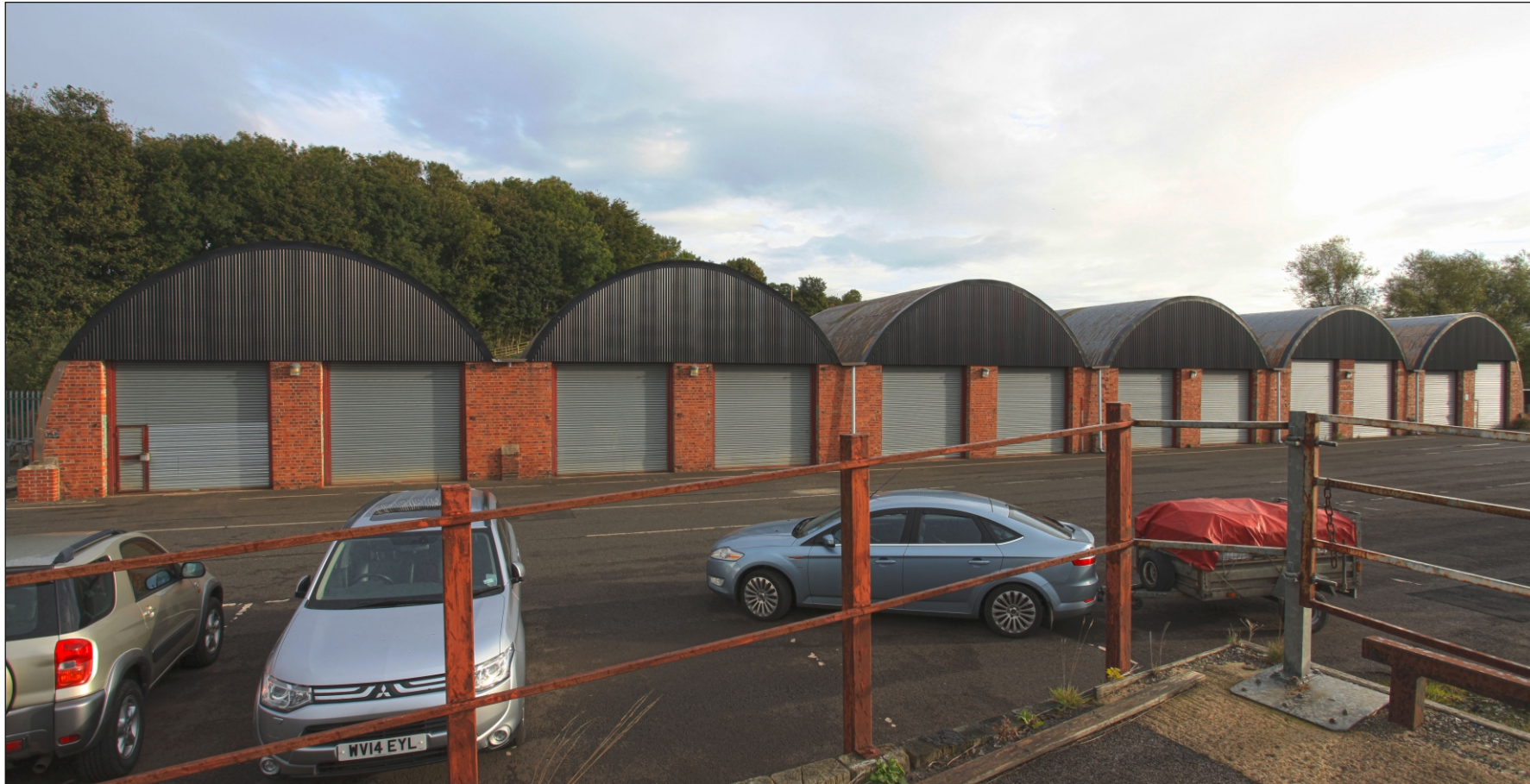
Plate 7: Oblique view of the south elevation of the tank garages (Romney sheds), looking north-east
