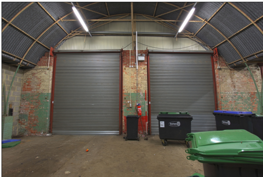
Plate 34: View of the south wall in G5, looking south
