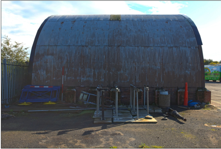
Plate 12: View of the west elevation of the tank garages (Romney sheds)
