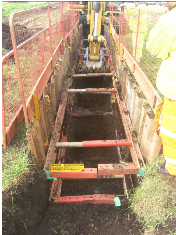
Plate 2: Service trench visibility, view from north
