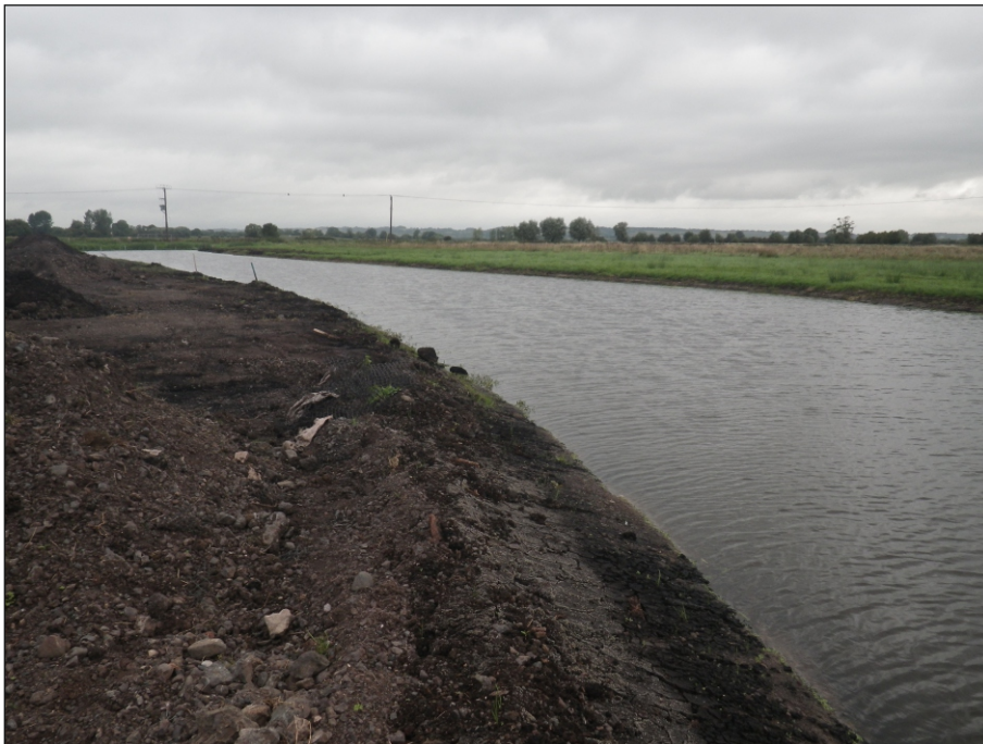
Plate 8: Newly flooded channel, south of road
