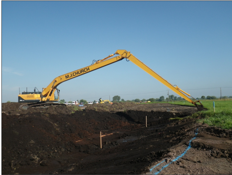
Plate 5: Channel excavation, south of road
