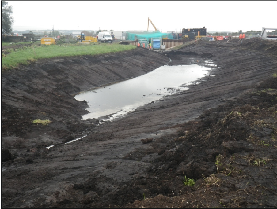
Plate 7: Excavated channel, north of road
