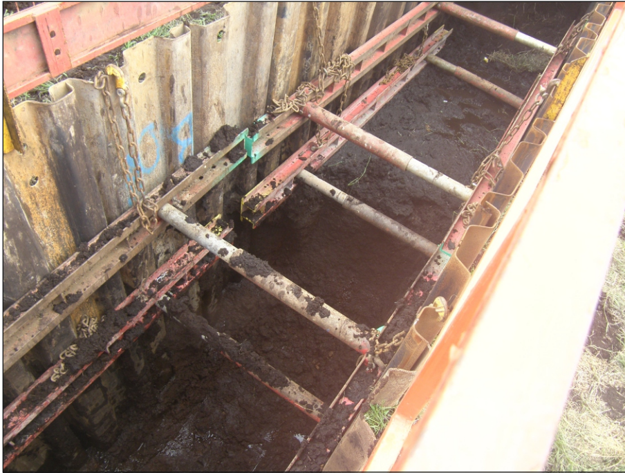
Plate 3: Service trench, view from north-west
