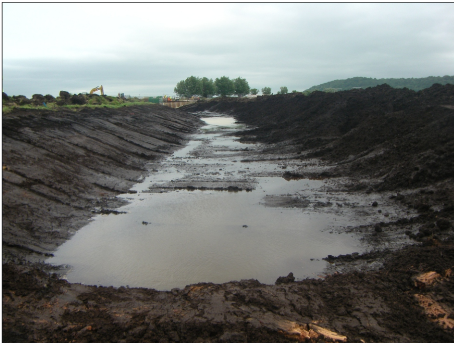
Plate 4: Excavated channel, north of road
