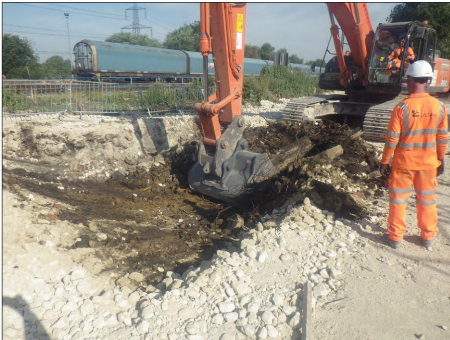
Plate 4: Working shot during watching brief
