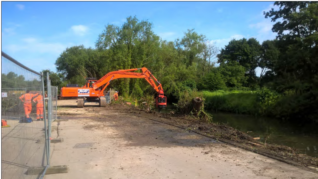
Plate 6: Working shot of piling during watching brief
