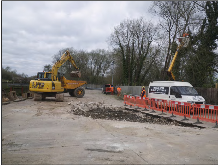
Plate 1: Working shot of machining the excavation area
