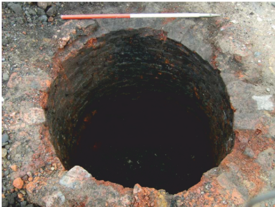
Plate 16: Brick superstructure of well 9136 with a wooden beam found in situ; looking vertical
