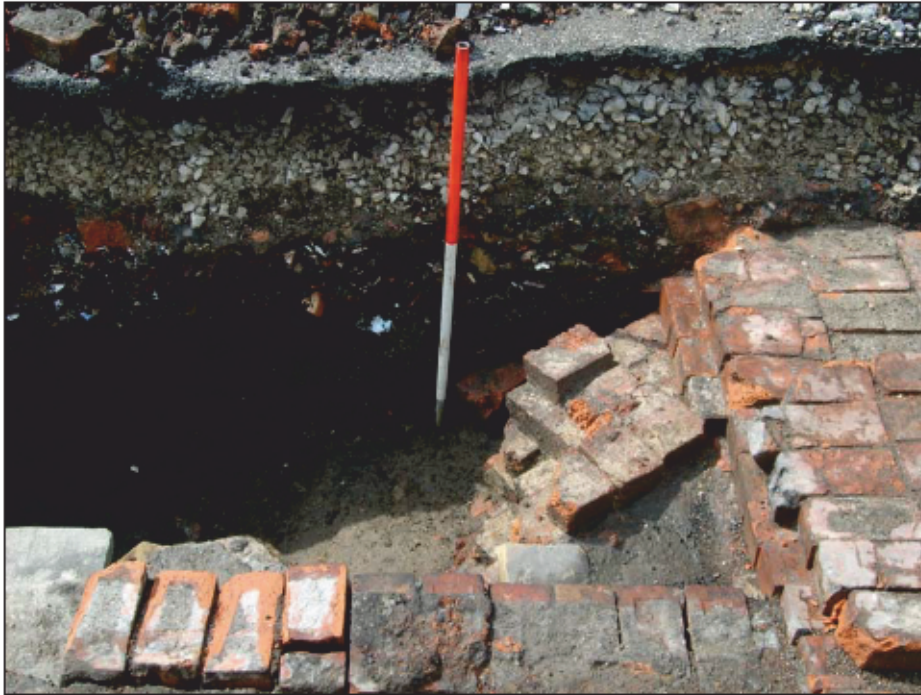
Plate 21: Demolition deposit 4012, hard core 4001 and tarmac 4000 of the car park; looking south
