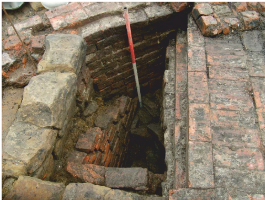
Plate 8: Hand-made brick walling 9208 truncated by wall 9045 and overlaid by sandstone wall 9107 and brick wall 9033; looking north-east
