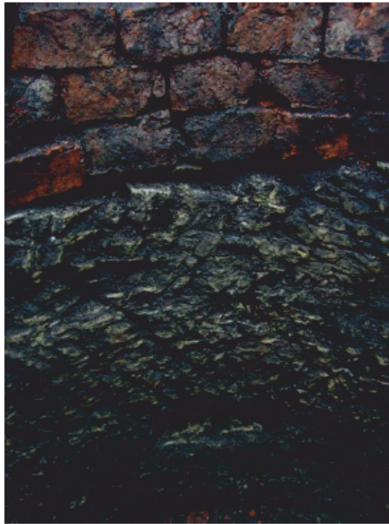
Plate 17: Details of construction of well 9136, including a step hole
