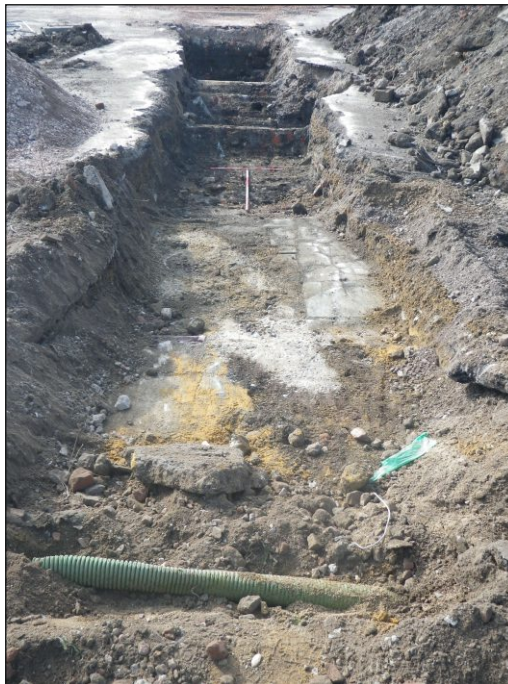
Plate 10: Paving and levelling/reclamation deposits in Trench 7, viewed from the north-east
