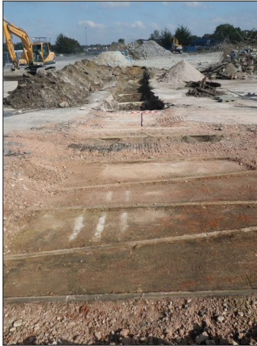
Plate 9: Tram/railway tracks in Trench 7, viewed from the south-west
