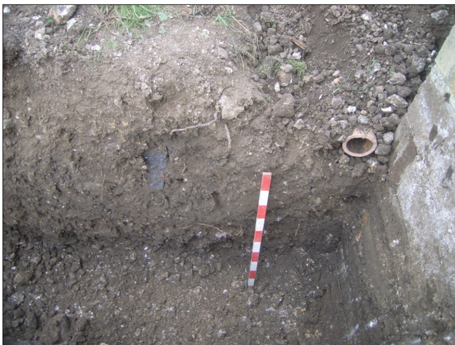
Plate 3: SW facing representative section in northernmost foundation trench showing disturbed soil directly overlying abundant flint gravel natural.
