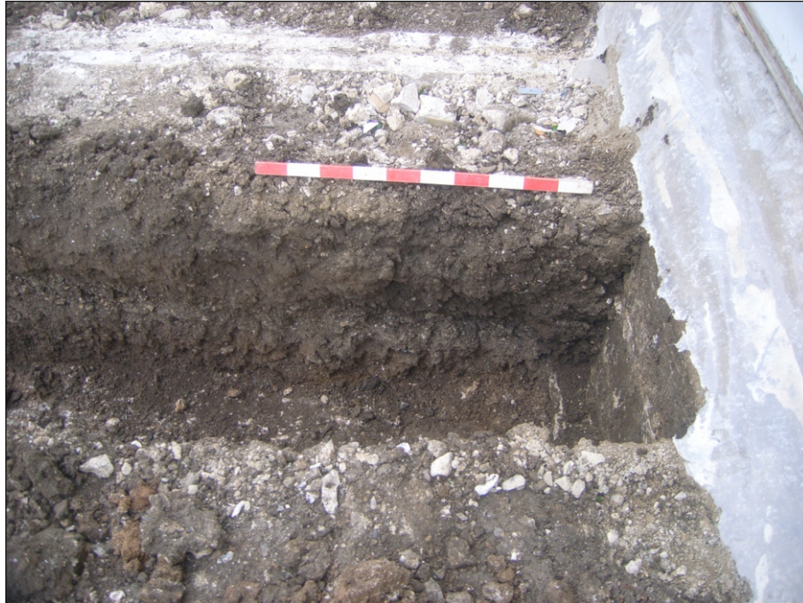
Plate 2: SW facing representative section in central foundation trench showing disturbed soil and foundation trench for existing wall above a silty layer with abundant small gravel (slightly stepped out in plate) over yellowish/reddish brown natural clay and degraded chalk.
