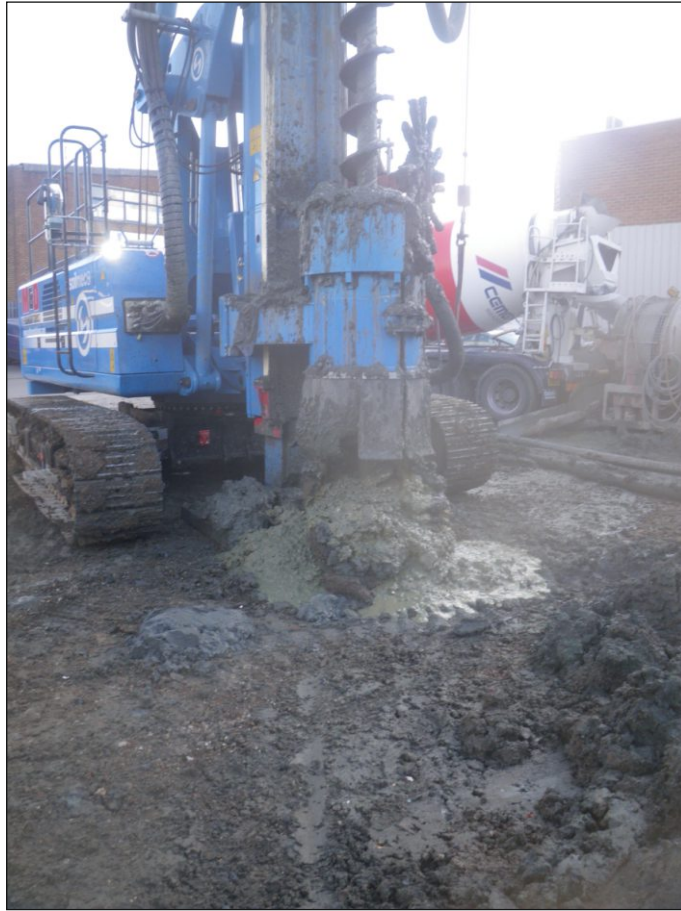
Plate 3: Typical pile hole in south-east of Site, looking south-east
