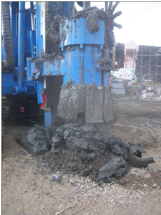
Plate 2: Typical pile hole in north-east of Site, looking west
