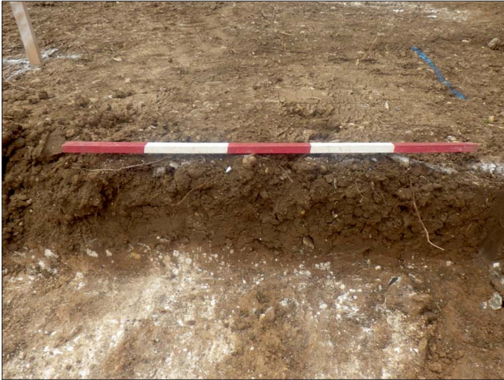
Plate 1: Representative section at south-western end of pipe trench, view from the north-west.
