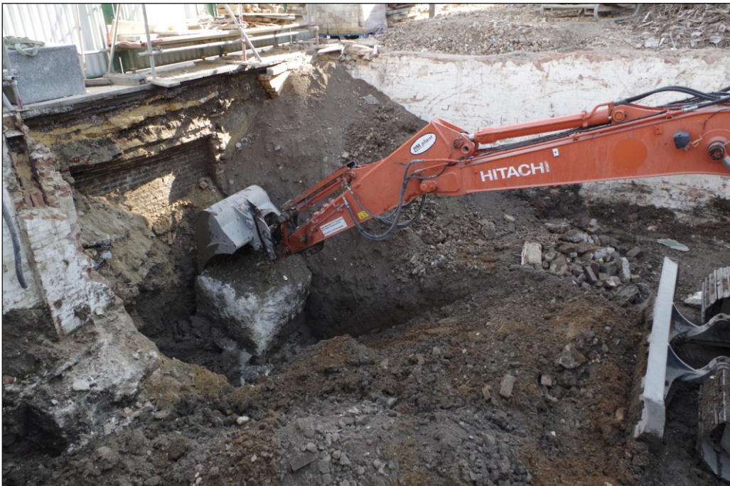
Plate 6: Working shot, removal of concrete slab
