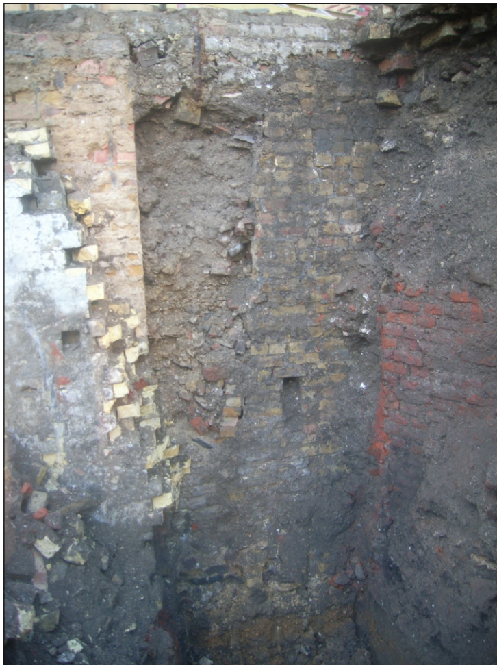
Plate 8: Retaining wall for neighbouring fire station
