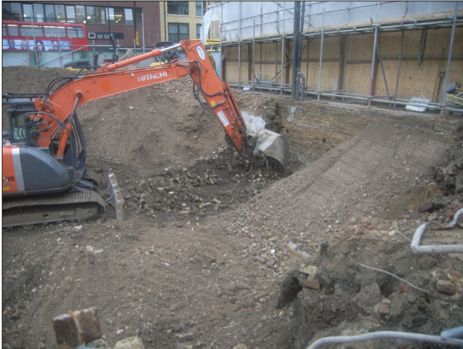
Plate 7: Working shot, removal of western retaining wall
