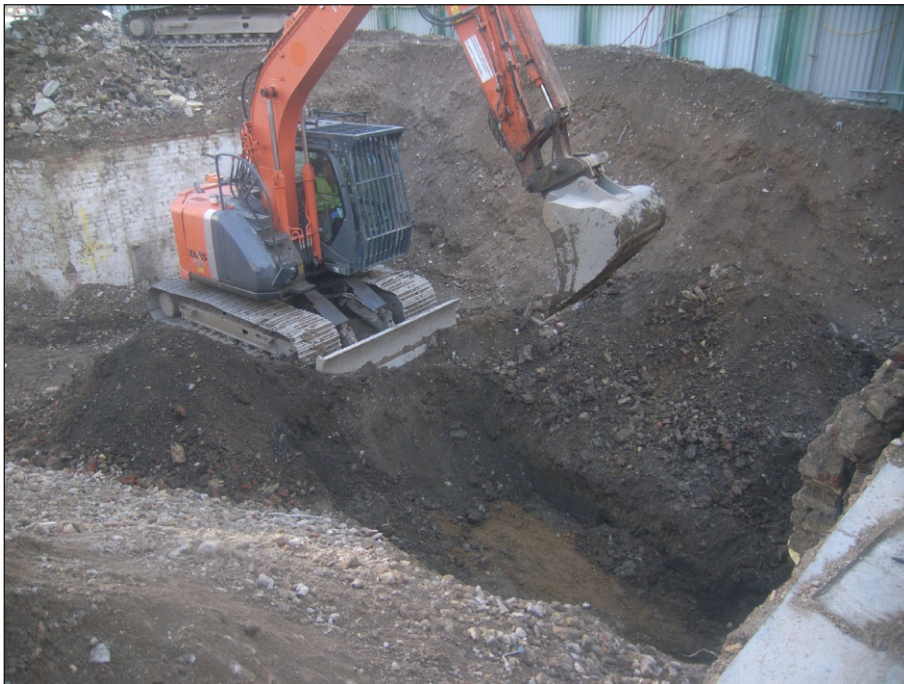
Plate 2: Working shot from the western wall
