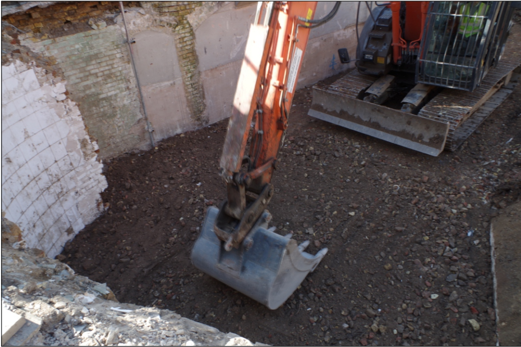
Plate 3: Backfilling of south east corner of the Site after probing
