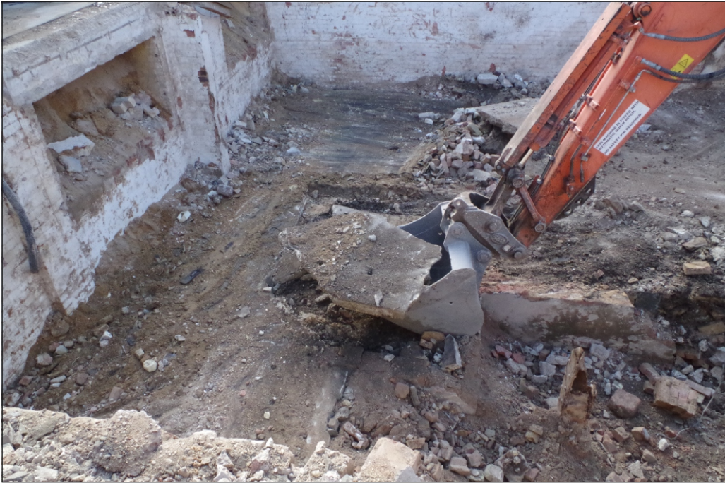
Plate 5: Working shot, removal of concrete floor
