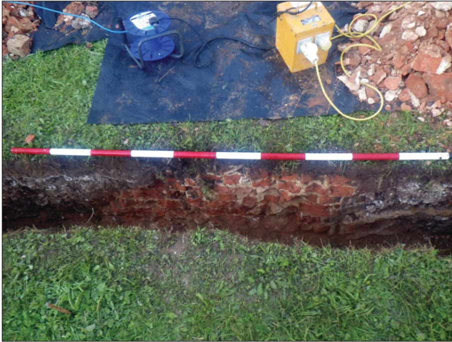
Plate 5: View from east of wall 407 in section (2 m scale)
