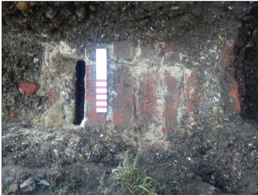
Plate 3: View from above of brick culvert drain 302 (0.2 m scale)
