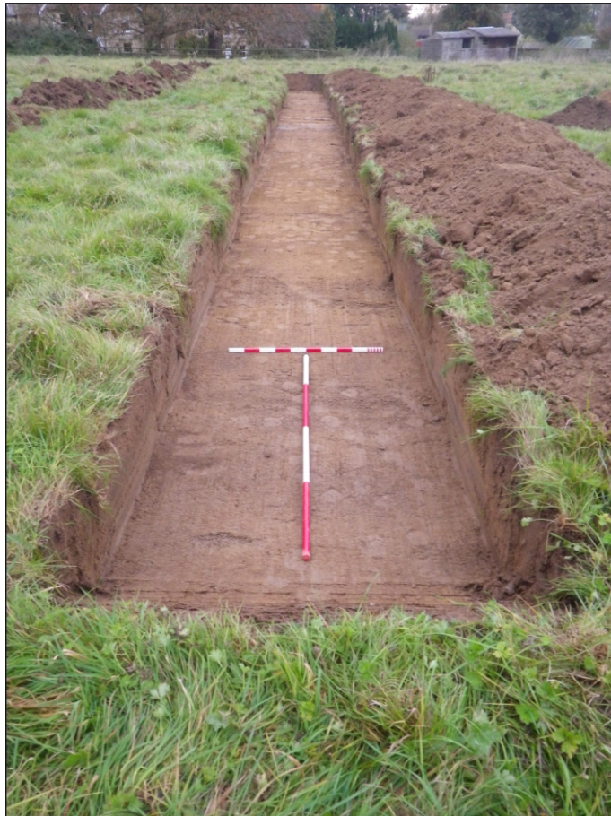
Plate 1: Trench 2 viewed from the south-west
