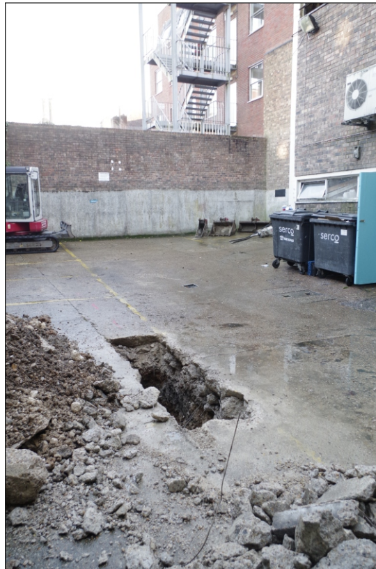
Plate 2: Location of Trench 1 – view from the north-west
