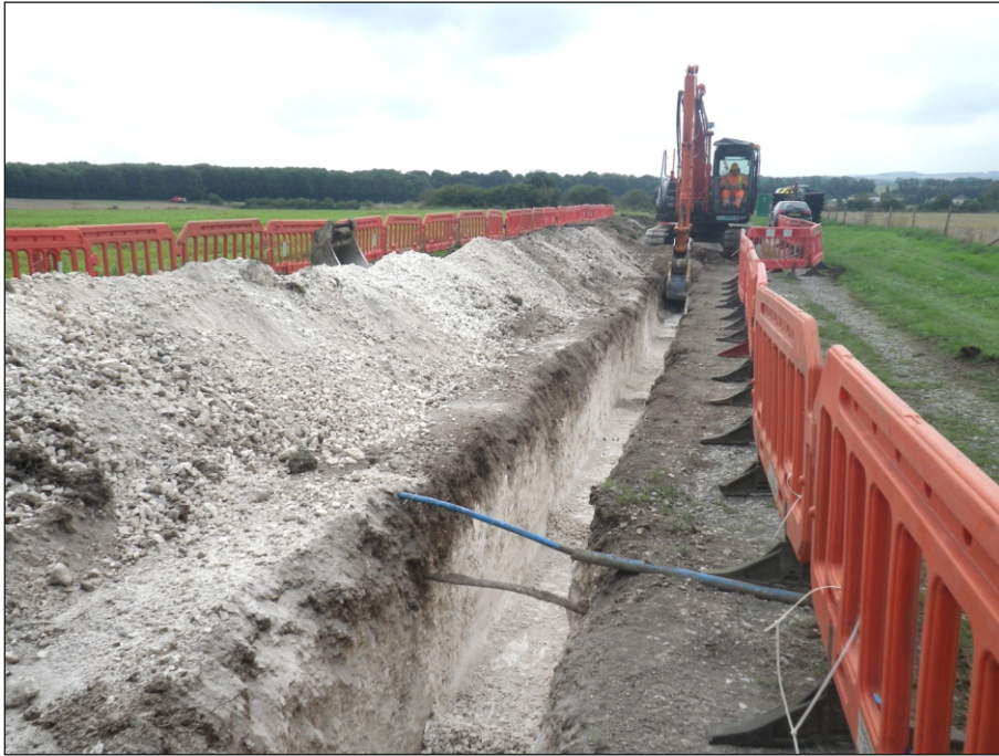
Plate 5: Working shot, Trench C-D
