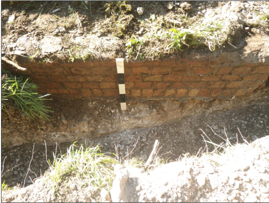
Plate 3: Wall 1049, north-facing elevation
