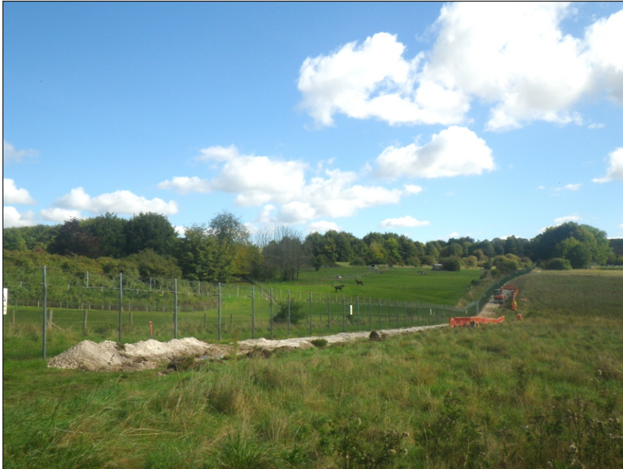
Plate 1: General view of Trench C-D taken from the south-west
