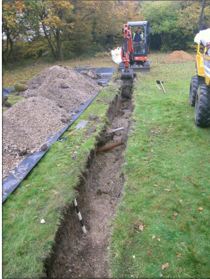
Plate 3: Drainage trench under excavation
