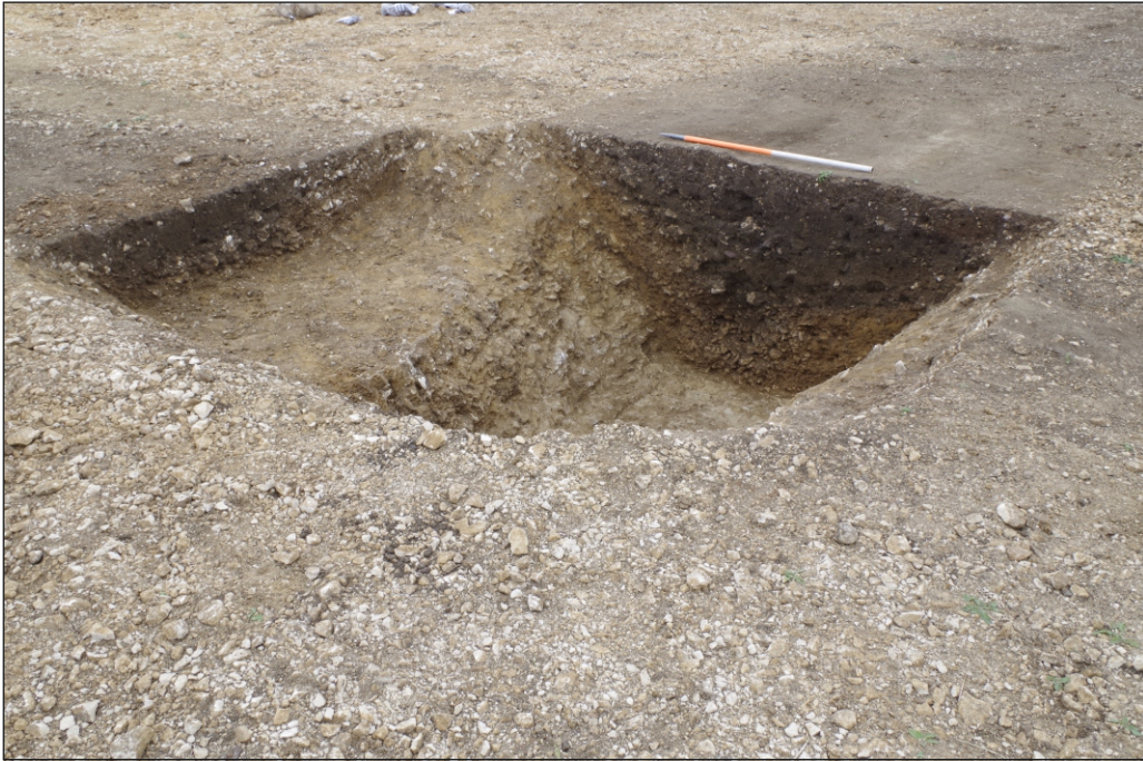
Plate 17: North-west corner of enclosure, facing south-east
